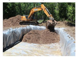
the water from your drainage tile through a trench filled with wood chips. Denitrifying bacteria in those wood chips can remove any nitrates in the water. Flat ground or sloping, and whatever soil you might have—this practice works wherever you want it to.
