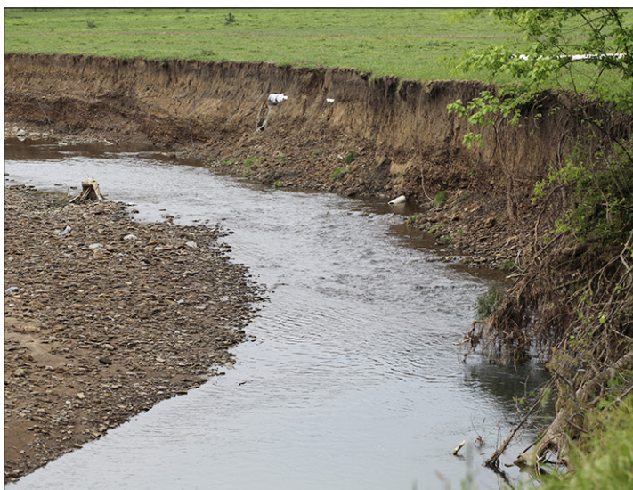
A recently completed Emergency Watershed Protection Program streambank stabilization project in Madison County protects a county water line and sewer line that run along Wharton Creek. (Left) Flooding in 2017 eroded the bank and exposed the water and sewer lines along with telecommunication cables. NRCS funded and designed the project and oversaw construction.
