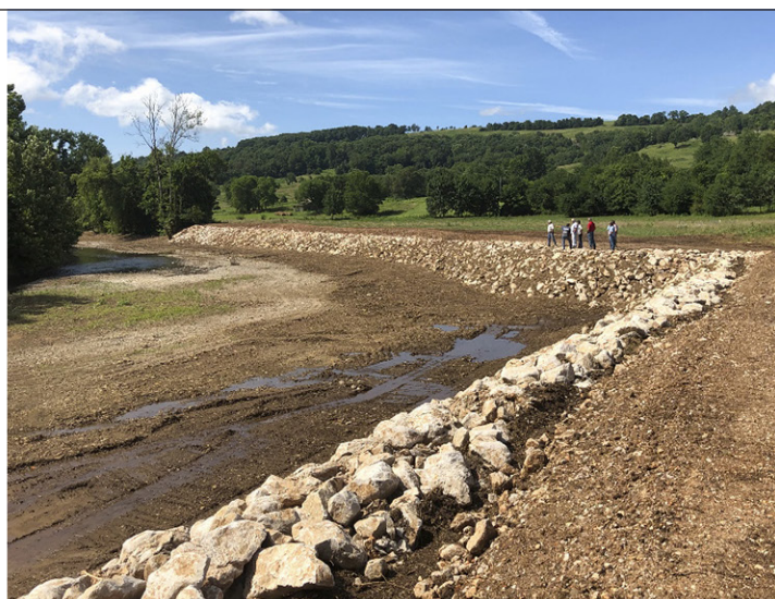
A recently completed Emergency Watershed Protection Program streambank stabilization project in Madison County protects a county water line and sewer line that run along Wharton Creek. (Left) Flooding in 2017 eroded the bank and exposed the water and sewer lines along with telecommunication cables. NRCS funded and designed the project and oversaw construction.
