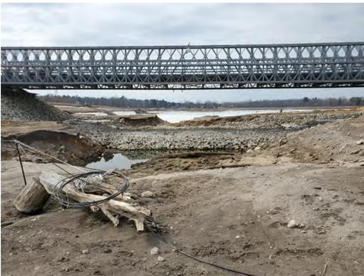
*(below) Over the winter, work continued on the Tobacco River spillway adjacent to the Edenville Dam. A concrete weir was constructed to lower Wixom Lake and restore the Tobacco River to its original course.*
