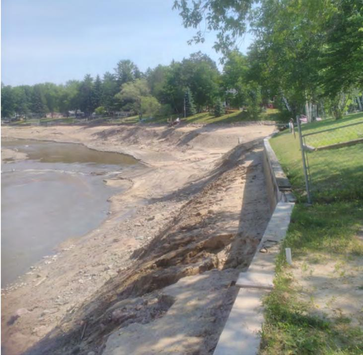
*(below) Streambank stabilization and slope stabilization work at the same site repaired the damage and protected the area from further erosion.*
