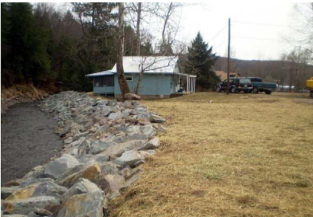
After: Through NRCS's Emergency Watershed Protection program, over 400 feet of rip rap was installed to protect the stream bank and prevent further erosion that could cause loss of life and property.
