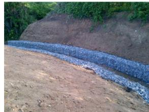
Open channel gabion outlet guard will keep the discharge area protected from runoff and erosion during rain events. (Photo: M. Rodriguez, NRCS)
