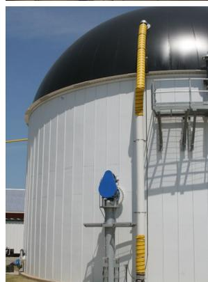
**Animal Waste Methane Digesters:** An anaerobic digester biologically treats agricultural waste to produce biogas (methane) used for energy production. The process also reduces odors, greenhouse gas emissions and pathogens.
