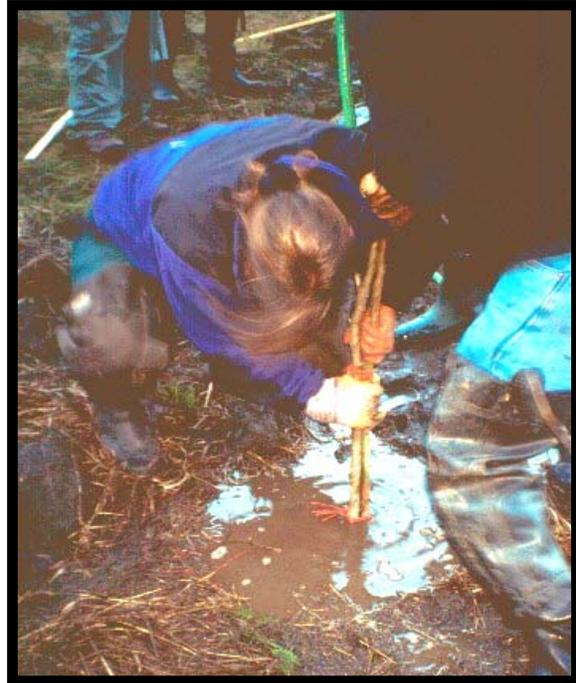
One problem that we have observed is that if there is a coarse soil layer under a layer of fine textured soil, when the waterjet drills into this coarse layer, the water in the hole will drain out into the coarse layer. This will defeat the purpose of planting the cuttings into slurry to eliminate air pockets. Pulling the waterjet nozzle up to just above the layer will allow sediment to settle back into the bottom of the hole and seal it again.
