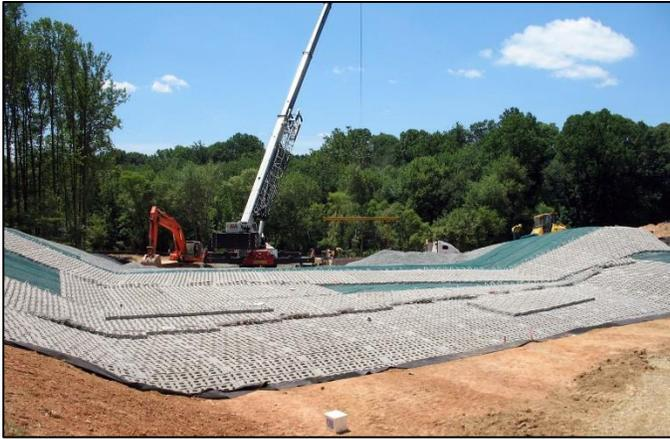
Articulated concrete blocks were installed to provide erosion control on the auxiliary spillway at Woodglen Lake.
