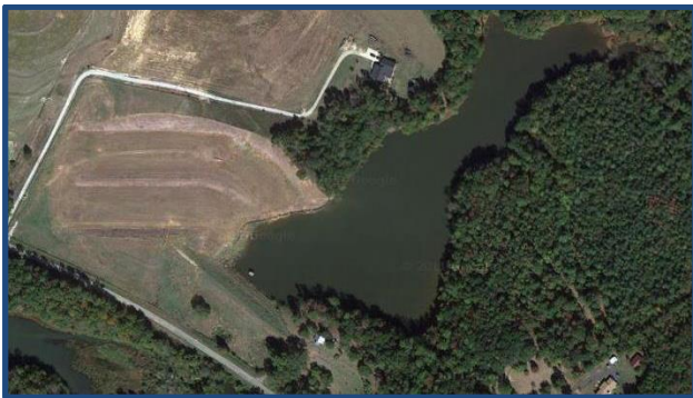
The rehabilitation project was completed in April 2012.
