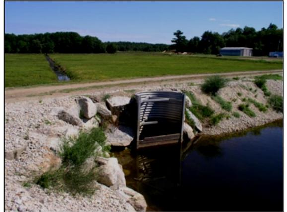
The structure may be part of a wildlife project that requires modification of the water flow with chutes or cold-water releases. Sluices to provide silt management; debris screens to keep trash, debris, or weed seeds out of pipelines; and tide gates to prevent backflow into a channel are examples of other uses of this practice. Bridges, culverts, flumes, inverted siphons, and long span pipes can be used to convey water over, under, or along a ditch, canal, road, railroad, or other barrier.
