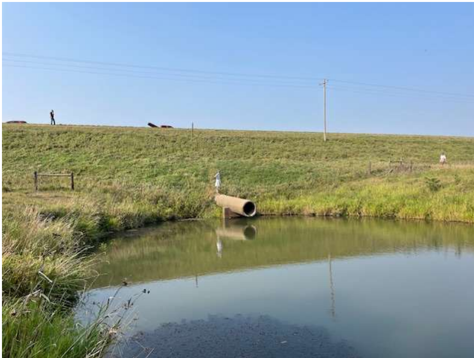
Plot 6b – Looking north from south side of dam on west side of outlet channel toward outlet structure pipe.
