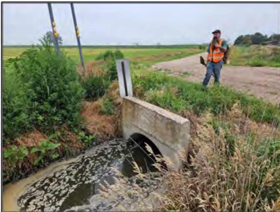
Figure 68. North Platte (Platte Valley) Canal: Feature 4 concrete culvert passing under the county road. Crew member for scale. View to the south-southeast. Photograph taken on July 21, 2025.
