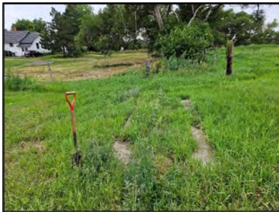
Figure 32. Site LN00-260. Feature 6 concrete foundation looking west. Shovel extending 3 ft above ground for scale. Photograph taken on July 18, 2025.
