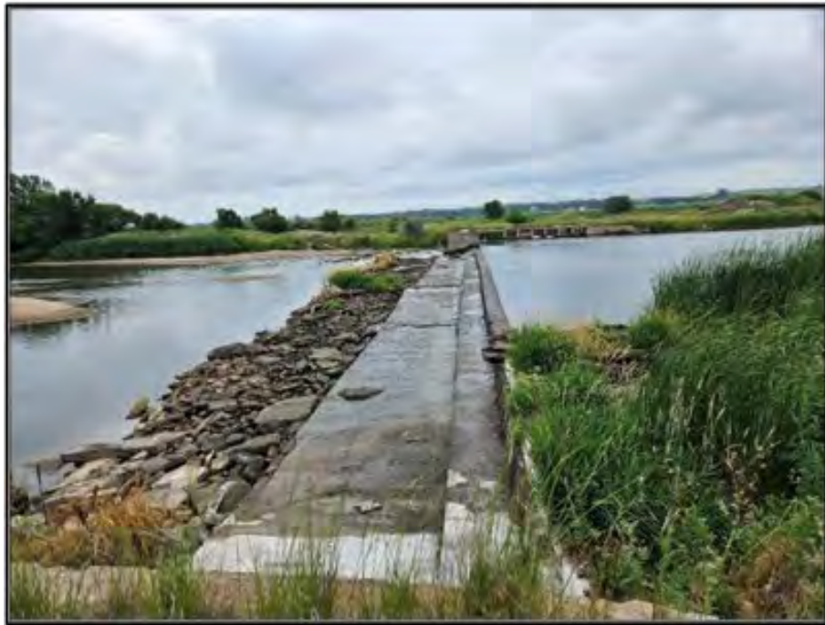
Figure 71. Paxton Hershey Canal: Feature 1, diversion dam overview looking southeast at the spillway apron and weir exposed while the water gates are open. Photograph taken on July 17, 2025.
