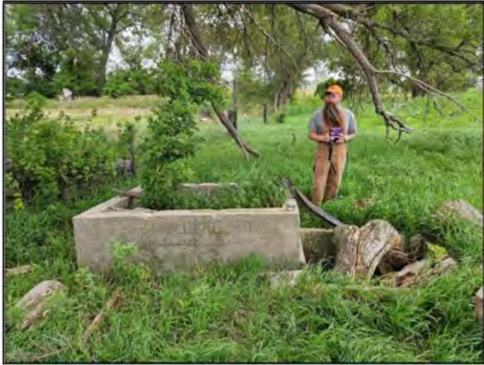
Figure 28. Site LN00-260. Feature 4 concrete water tank and pump house foundation overview looking west with crew member for scale. Photograph taken on July 18, 2025.
