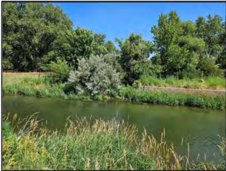
Figure 52. Keith Lincoln Canal: Feature 1 the overgrown return gate. View to the north.. Photograph taken on July 15, 2025.
