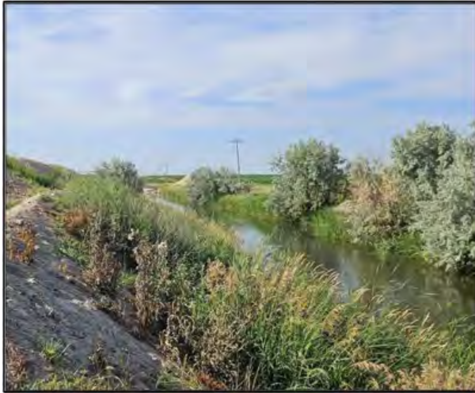
Figure 87. Suburban Canal: channel overview looking south. Photograph taken on July 19, 2025.
