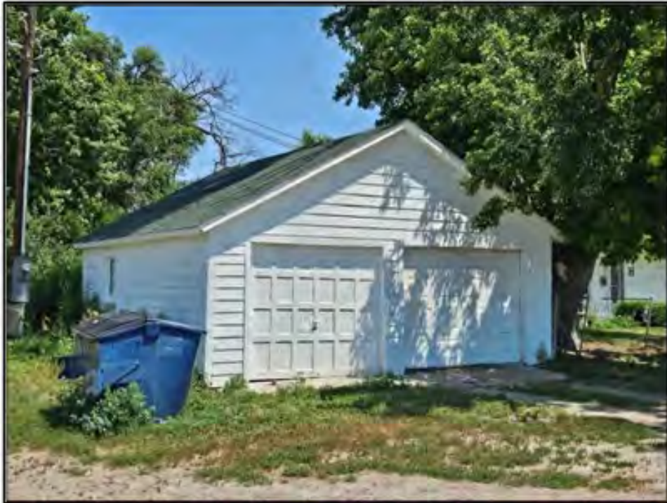
Figure 39. Site LN00-261. Feature 6 automobile garage looking northeast at the south and west elevations. Photograph taken on July 18, 2025.
