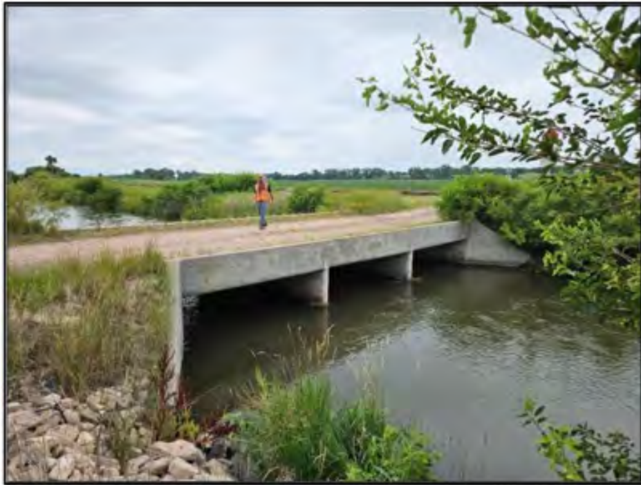
Figure 64. North Platte (Platte Valley) Canal: Feature 3 concrete vehicle bridge built in 1991 with crew member for scale. View to the east. Photograph taken on July 16, 2025.
