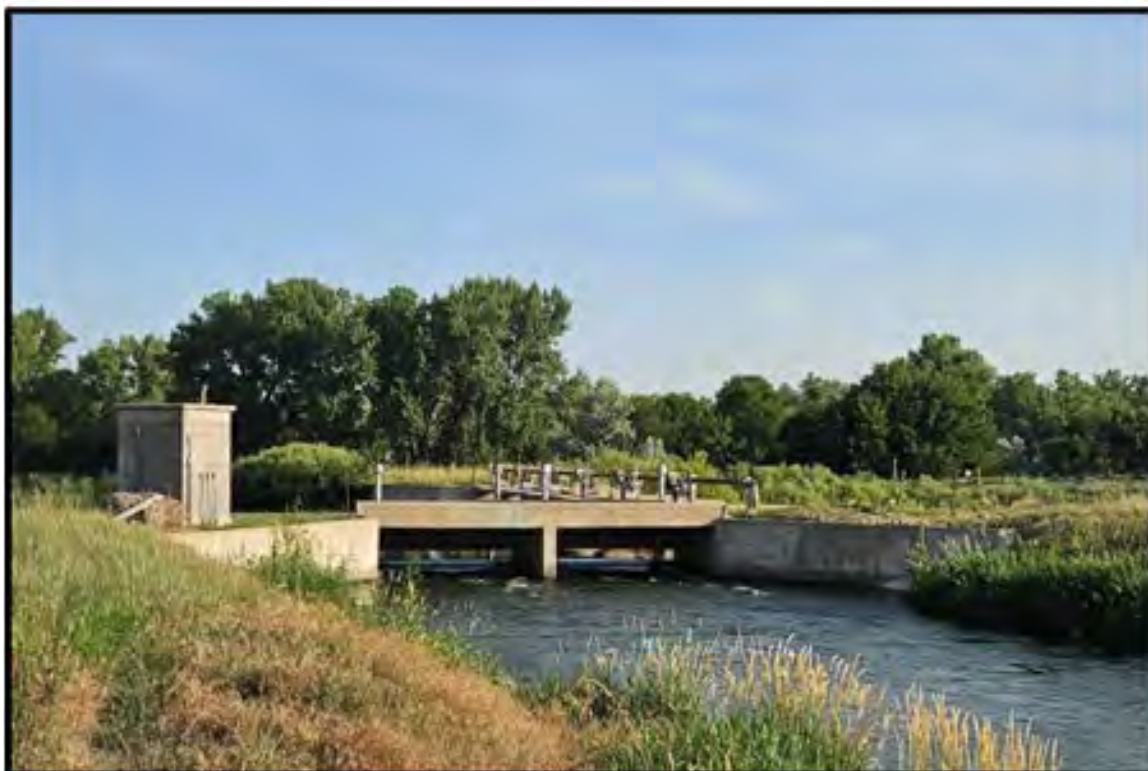
Figure 56. Keith Lincoln Canal: Feature 5, headgate. View to the north. Photograph taken on July 15, 2025.
