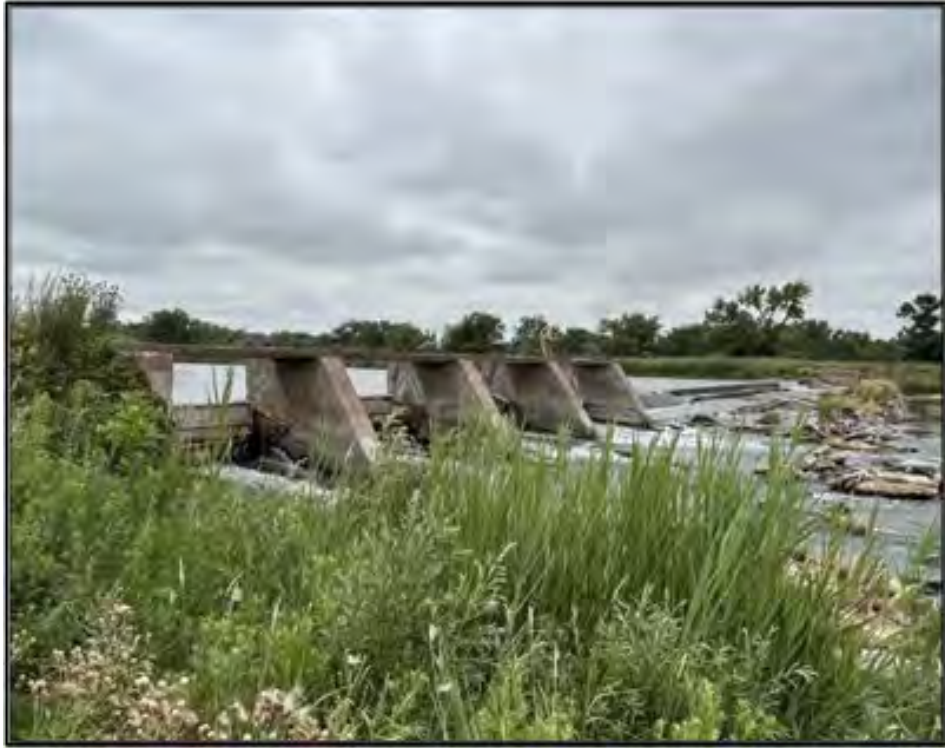
Figure 70. Paxton Hershey Canal: Feature 1, diversion dam overview looking southwest. Photograph taken on July 17, 2025.
