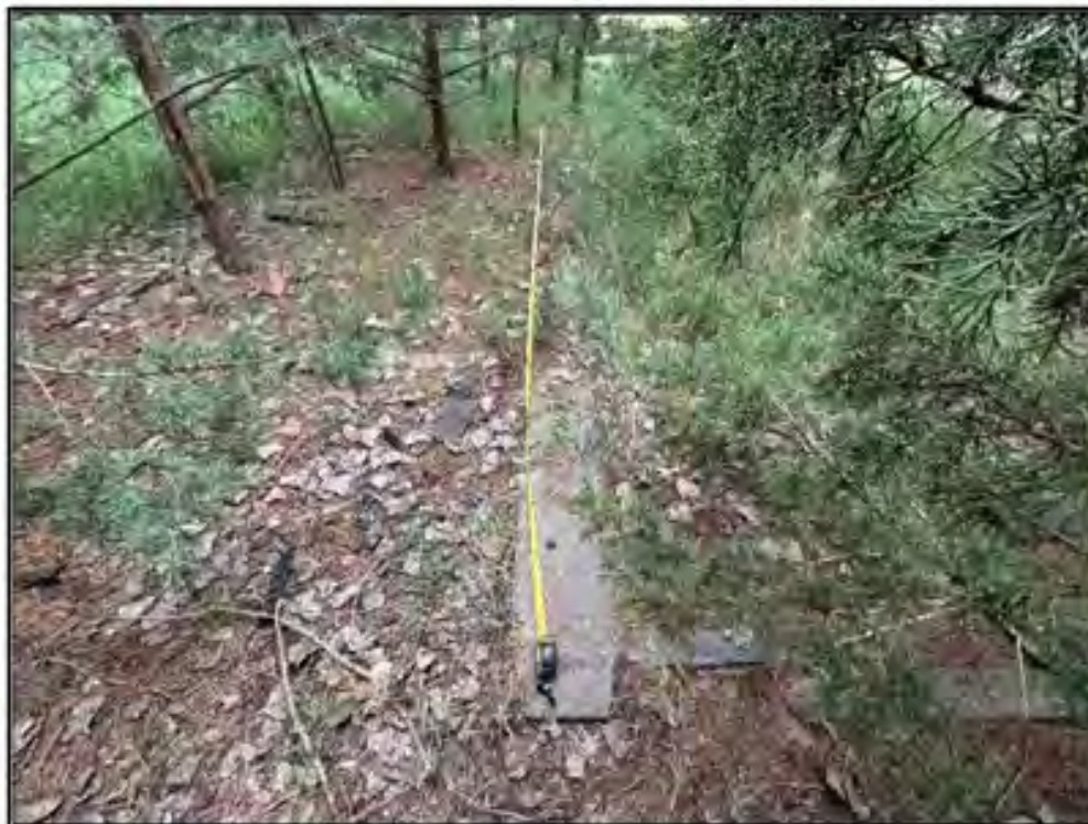
Figure 17. Site 25LN148. Feature 1 house foundation. View to the south from the northeast corner. Tape measure extended to 100 inches (8 ft 4 inches) for scale. Photograph taken by Derrick Maurer on July 16, 2025.
