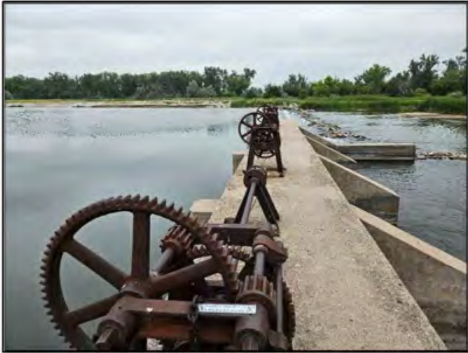
Figure 63. North Platte (Platte Valley) Canal: Feature 2 diversion dam, looking north along the top of the access platform with the hand operated gate equipment mounted on the platform. Photograph taken on July 16, 2025.
