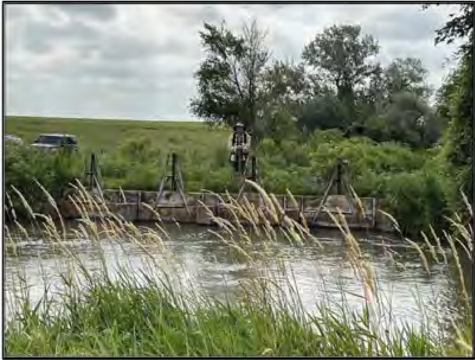
Figure 85. Birdwood Canal: Feature 2, headgate with crew member for scale. View to the south. Photograph taken on July 18, 2025.
