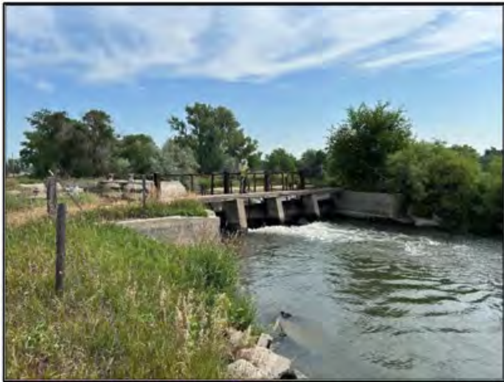
Figure 89. Suburban Canal: Feature 1, headgate with crew member for scale. View to the north. Photograph taken on July 19, 2025.
