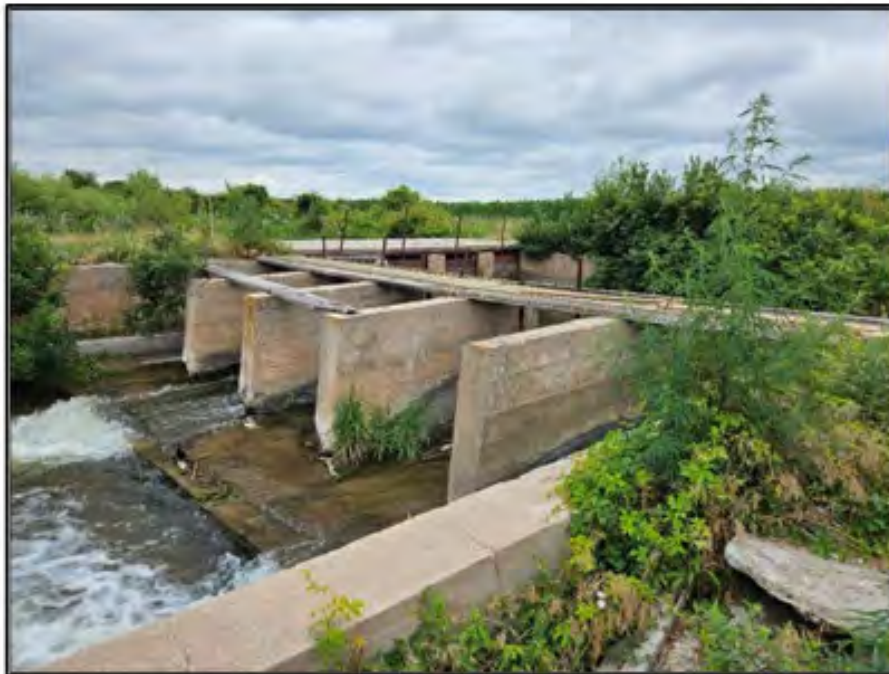
Figure 73. Paxton Hershey Canal: Feature 3 return channel gate, looking east. Photograph taken on July 17, 2025.
