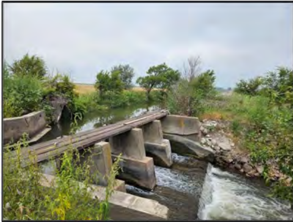
Figure 97. Cody Dillon Canal: Feature 3 return gate, looking southwest towards the canal channel. Photograph taken on July 21, 2025.
