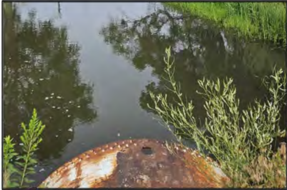
Figure 95. Cody Dillon Canal: Example of the riveted steel tank repurposed as a culvert at Feature 2 the culvert and sediment road crossing. View to the west. Photograph taken on July 21, 2025.
