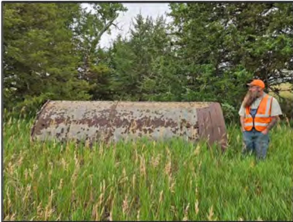
Figure 66. North Platte (Platte Valley) Canal: FS2, discarded radial gate with crew member for scale. View to the south. Photograph taken on July 16, 2025.
