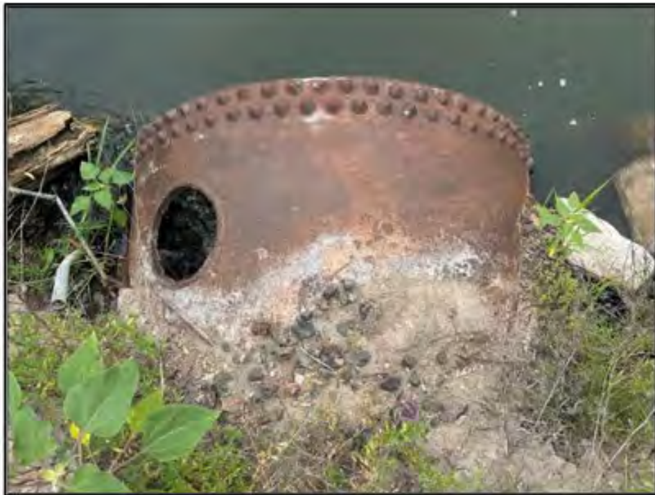
Figure 78. Paxton Hershey Canal: Example of the riveted steel tanks repurposed as culverts at Feature 6 the culvert and sediment road crossing. View to the east. Photograph taken on July 17, 2025.
