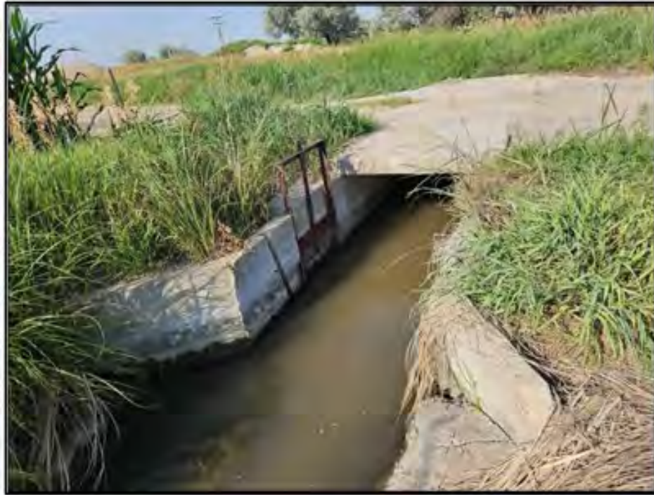
Figure 82. Paxton Hershey Canal: Feature 10, concrete box culvert. View to the west. Photograph taken on July 19, 2025.
