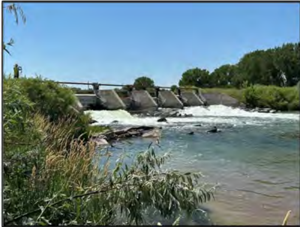
Figure 58. Keith Lincoln Canal: Feature 6, diversion dam overview. View to the southwest. Photograph taken on July 15, 2025.
