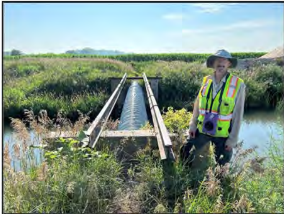
Figure 81. Paxton Hershey Canal: Feature 9, the corrugated steel flume allowing the Paxton Hershey Canal to pass over the Suburban canal. Crew member for scale. Photograph taken on July 19, 2025.
