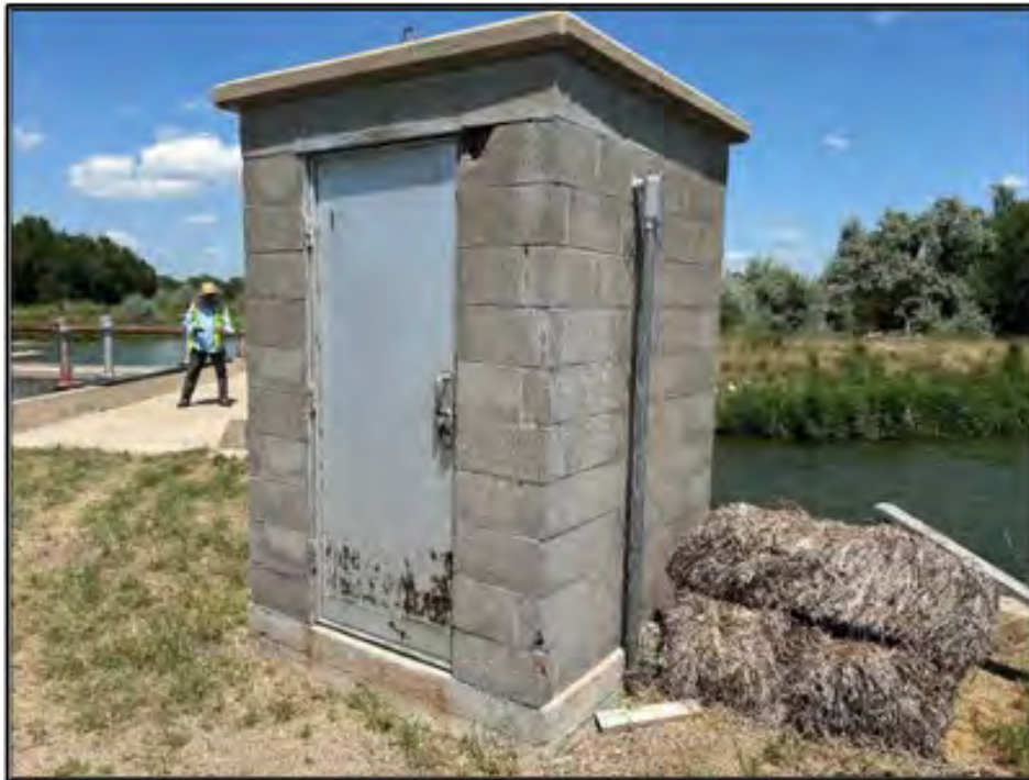
Figure 55. Keith Lincoln Canal: Feature 4, the diversion dam control shed. View to the north. Photograph taken on July 15, 2025.
