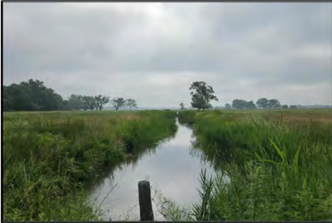
Figure 93. Cody Dillon Canal: channel overview looking east from a culvert road crossing of the canal (Feature 2). Photograph taken on July 21, 2025.
