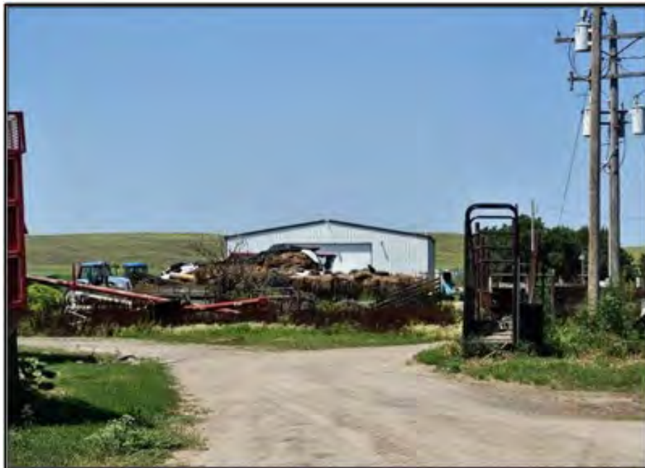
Figure 44. Site LN00-261. Feature 13, modern steel machine shed and storage building looking west at the east elevation. Photograph taken on July 18, 2025.
