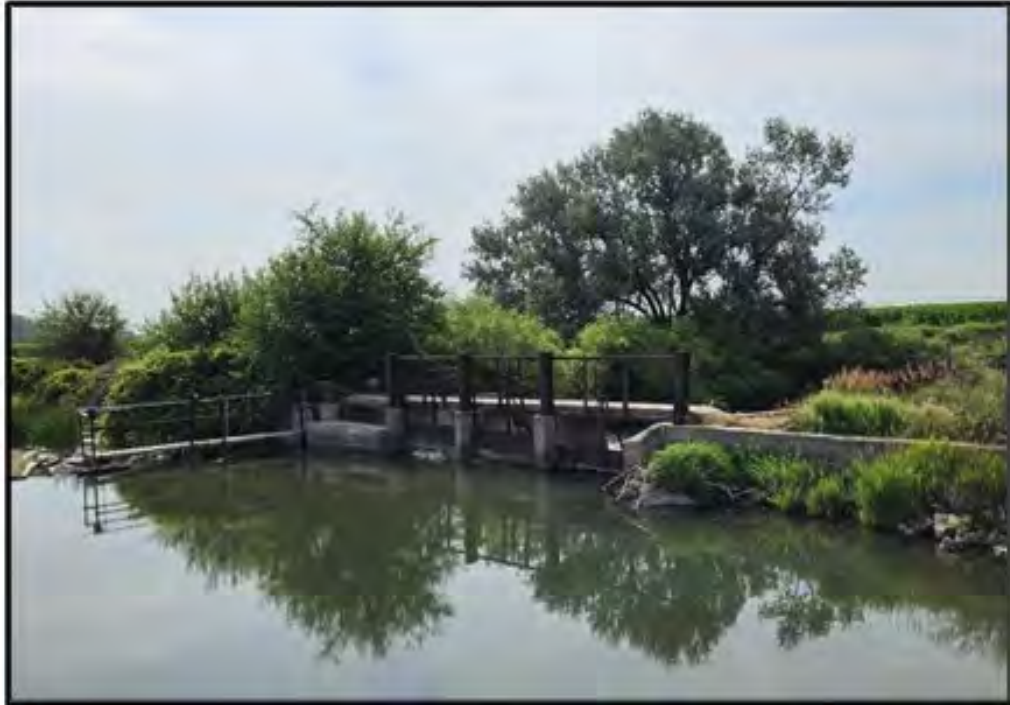
Figure 88. Suburban Canal: Feature 1, headgate. View to the southeast. Photograph taken on July 19, 2025.
