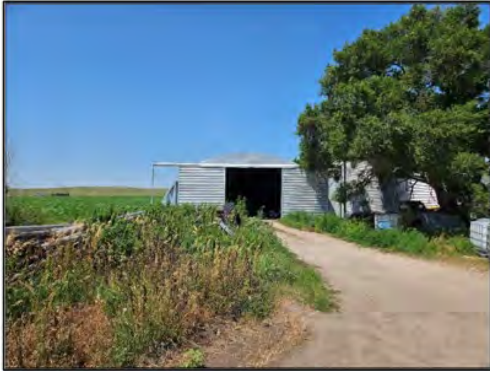
Figure 43. Site LN00-261. Feature 12, modern steel Quonset storage building looking west at the east elevation. Photograph taken on July 18, 2025.
