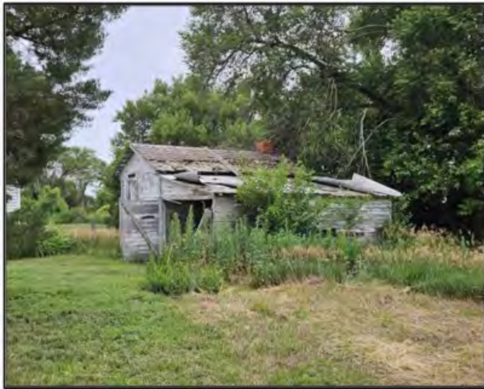
Figure 27. LN00-260. Feature 3 summer kitchen and lean-to addition, facing southwest toward the north and east elevations. Photograph taken on July 18, 2025.
