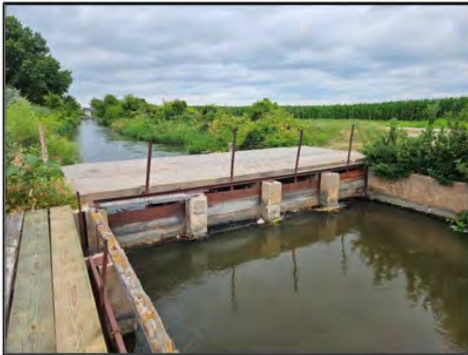
Figure 74. Paxton Hershey Canal: Feature 4, mid-channel gate capped by a concrete vehicle bridge deck. View to the east-northeast. Photograph taken on July 17, 2025.
