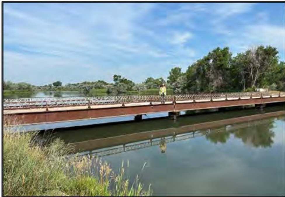
Figure 49. Site KH00-104. Overview of the bridge looking northwest with crew member for scale. Photograph taken on July 19, 2025.
