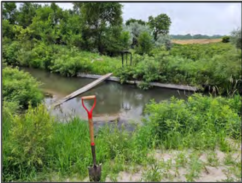
Figure 86. Birdwood Canal: Feature 3, disused rating flume. View to the southwest. Shovel extending 3 ft above ground for scale. Photograph taken on July 18, 2025.
