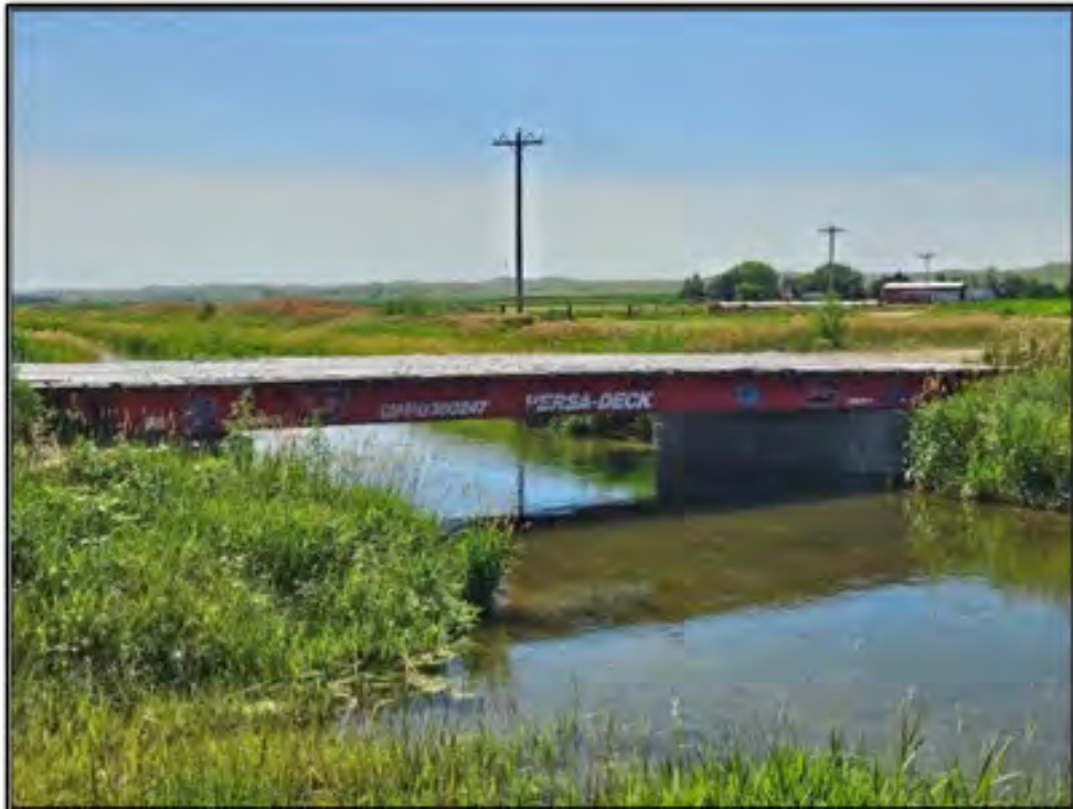
Figure 54. Keith Lincoln Canal: Feature 3, modern vehicle bridge. View to the southeast. Photograph taken on July 15, 2025.
