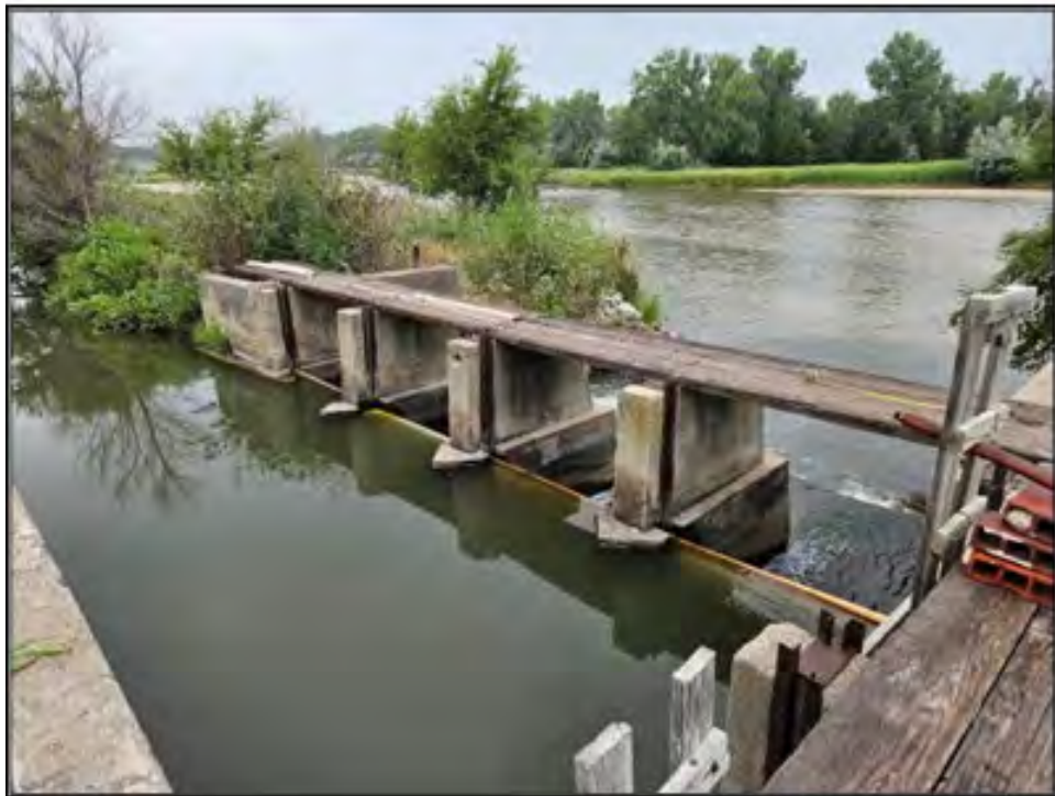
Figure 96. Cody Dillon Canal: Feature 3 return gate, looking northwest towards the North Platte River. Photograph taken on July 21, 2025.
