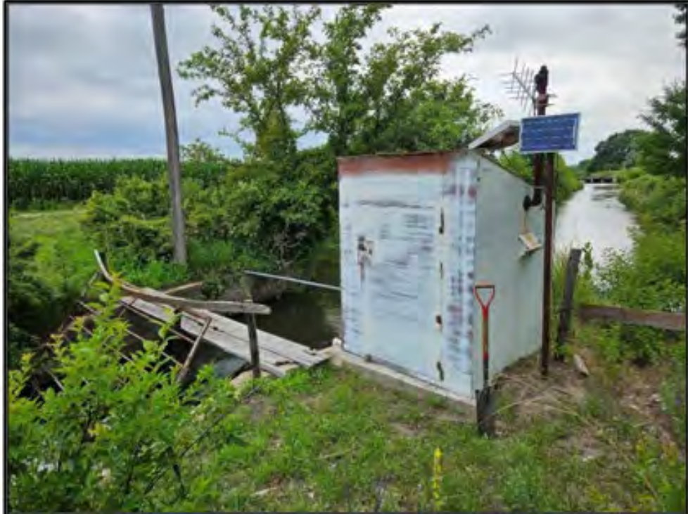
Figure 75. Paxton Hershey Canal: Feature 5 gaging station and fall structure. View to the southwest. Shovel extending 3 ft above ground for scale. Photograph taken on July 17, 2025.
