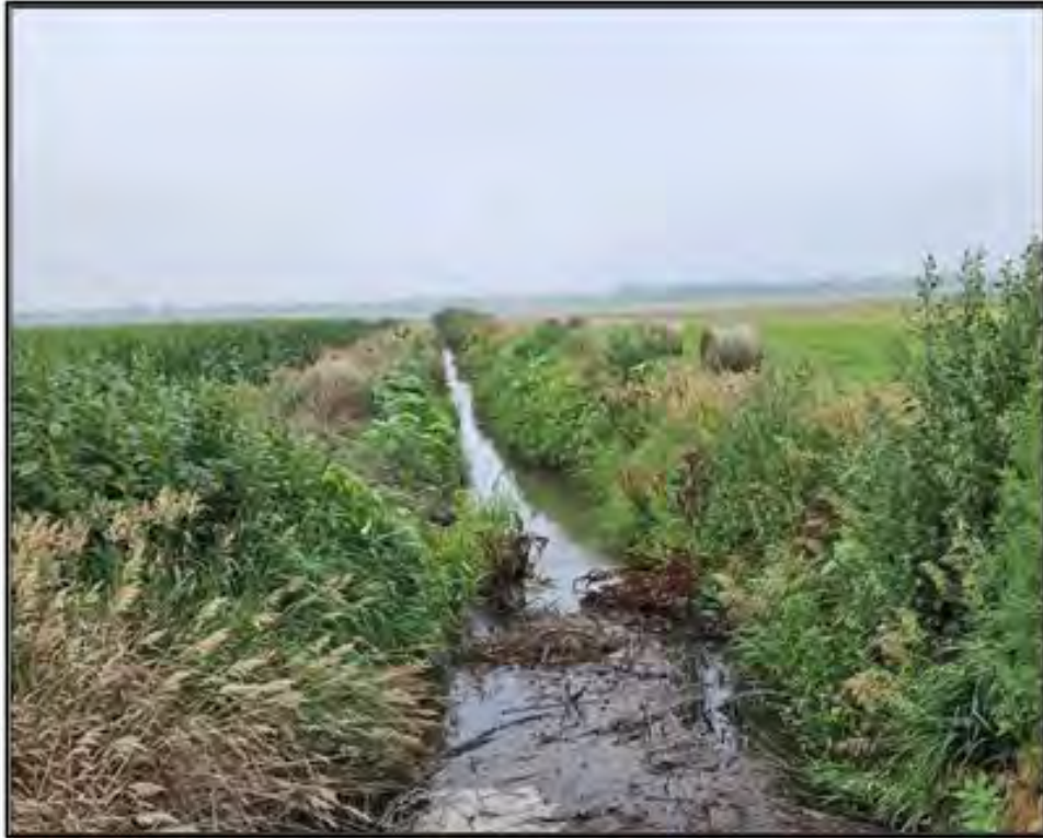
Figure 67. North Platte (Platte Valley) Canal: channel overview, Segment 2 return channel. View to the north. Photograph taken on July 21, 2025.
