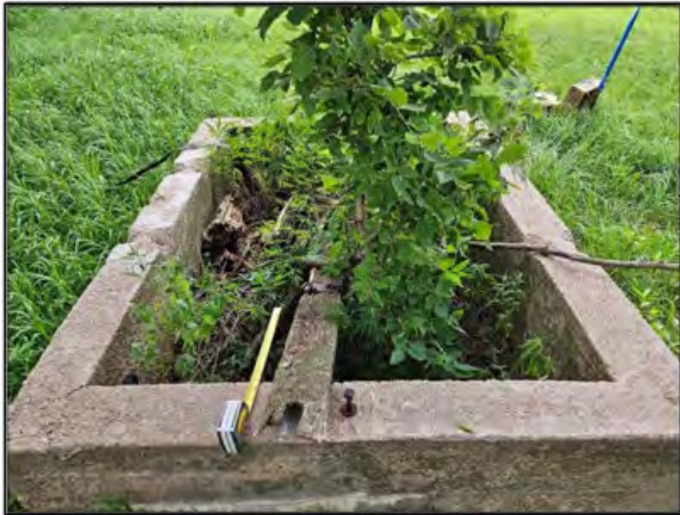
Figure 29. Site LN00-260. Feature 4 concrete water tank detail view looking north. Tape measure extended to 15 inches for scale. Photograph taken on July 18, 2025.
