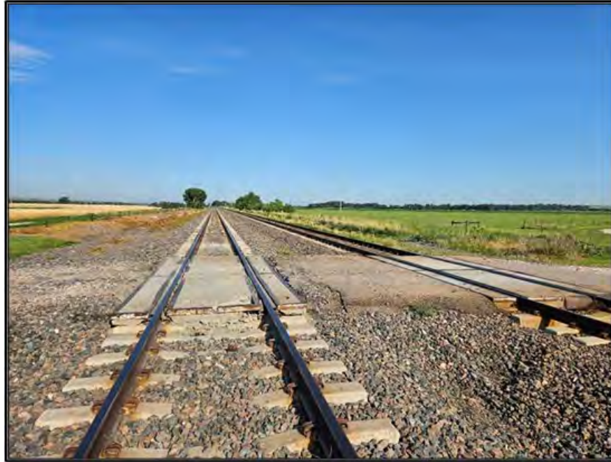
Figure 100. O&RV / Union Pacific Railroad: Segment 1 overview at the north end of the Keith Lincoln access road corridor survey area. View to the west. Photograph taken on July 15, 2025.
