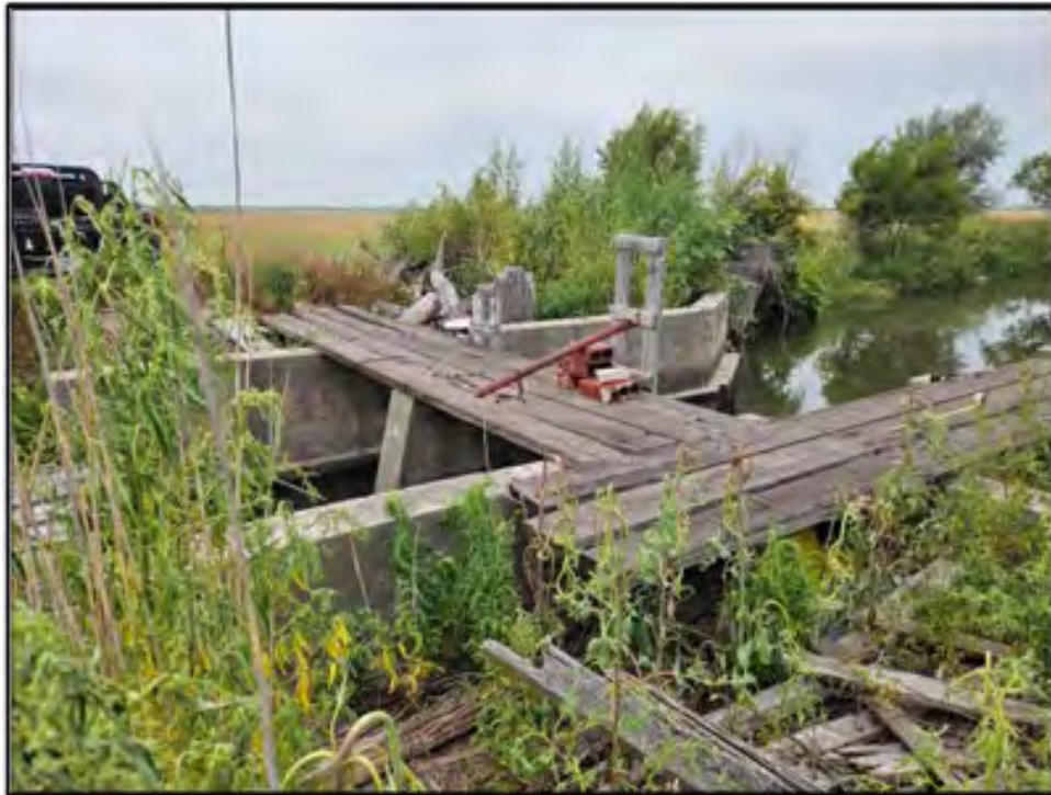
Figure 98. Cody Dillon Canal: Feature 4 headgate. View to the south. Photograph taken on July 21, 2025.
