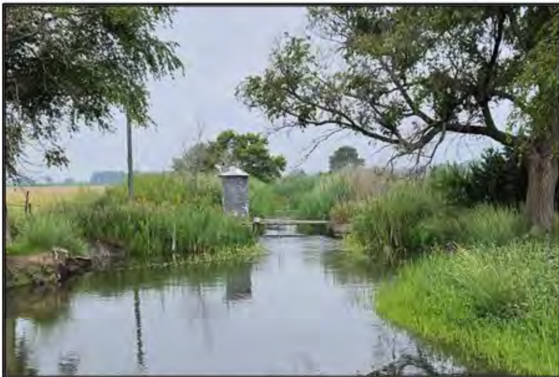
Figure 94. Cody Dillon Canal: Feature 1, gaging station. View to the west. Photograph taken on July 21, 2025.
