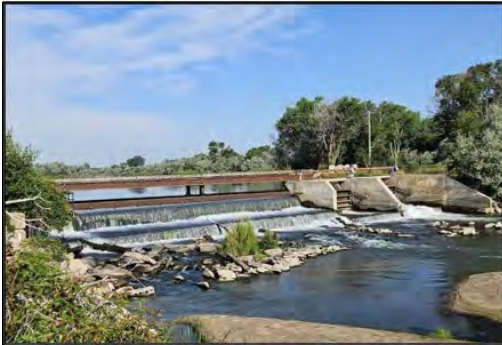
Figure 90. Suburban Canal: Feature 2, diversion dam. View to the west. Photograph taken on July 19, 2025.
