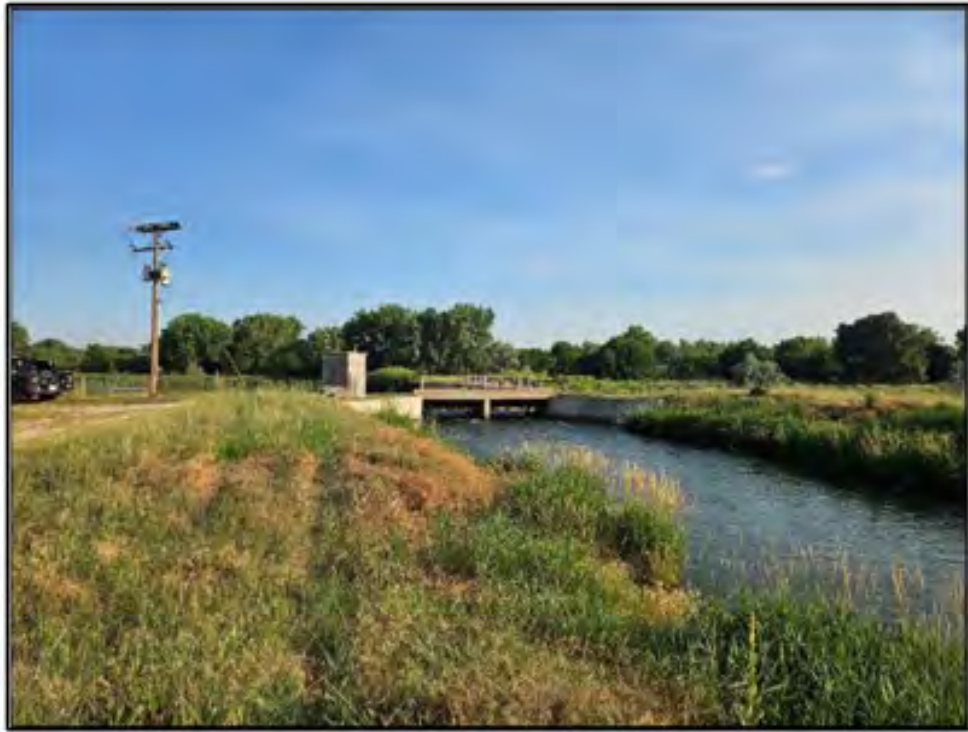
Figure 51. Keith Lincoln Canal: channel overview looking northwest towards the headgate (Feature 5). Photograph taken on July 15, 2025.
