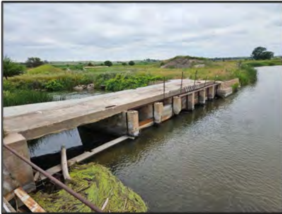
Figure 72. Paxton Hershey Canal: Feature 2 headgate, looking southeast. Photograph taken on July 17, 2025.
