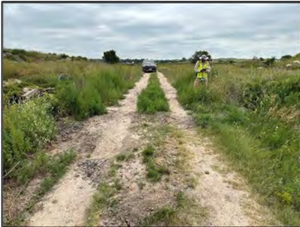
Figure 77. Paxton Hershey Canal: Feature 6 the culvert and sediment road crossing. View to the southeast with crew member for scale. Photograph taken on July 17, 2025.
