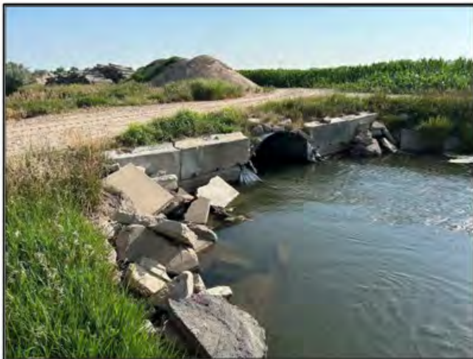
Figure 91. Suburban Canal: Feature 3, culvert and concrete retaining wall access road crossing. View to the northeast. Photograph taken on July 19, 2025.
