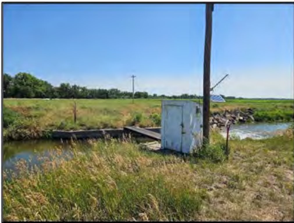
Figure 53. Keith Lincoln Canal: Feature 2, gaging station. View to the north. Photograph taken on July 15, 2025.
