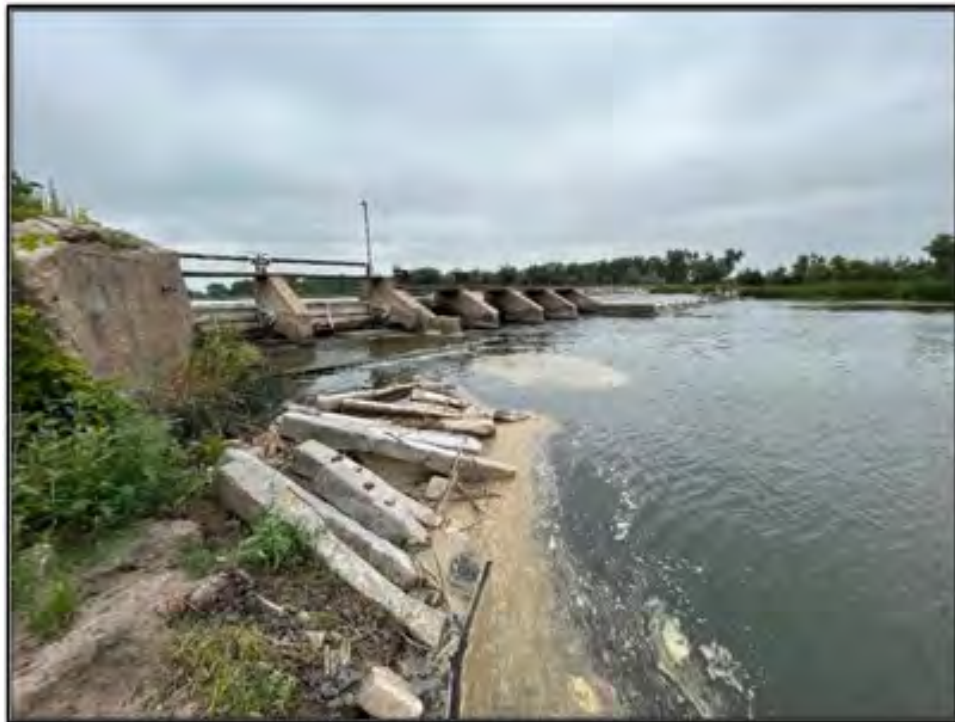
Figure 62. North Platte (Platte Valley) Canal: Feature 2 diversion dam overview, looking west. Photograph taken on July 16, 2025.
