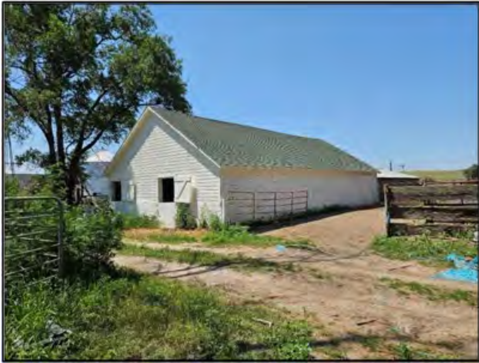
Figure 41. Site LN00-261. Feature 8 livestock barn looking southwest at the north and east elevations. Note Feature 9 to the right of the livestock barn. Photograph taken on July 18, 2025.
