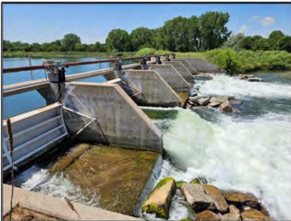
Figure 59. Keith Lincoln Canal: Feature 6, diversion dam radial water gates and access platform with crew member for scale. View to the northwest. Photograph taken on July 15, 2025.
