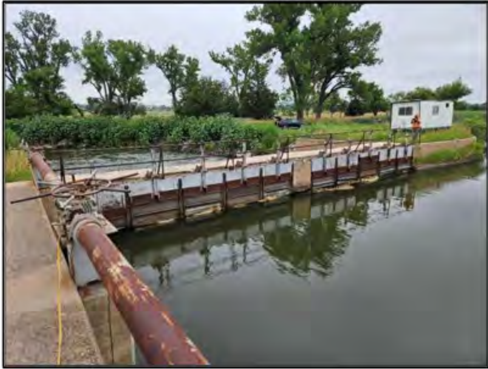
Figure 61. North Platte (Platte Valley) Canal: Feature 1 headgate, looking south. Photograph taken on July 16, 2025.
