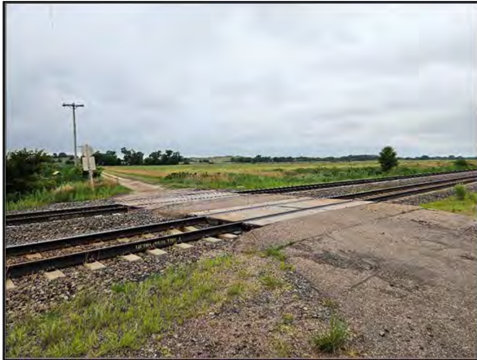
Figure 101. O&RV / Union Pacific Railroad: Segment 2, overview at the south end of the North Platte / Platte Valley access road corridor. View to the southwest. Photograph taken on July 16, 2025.
