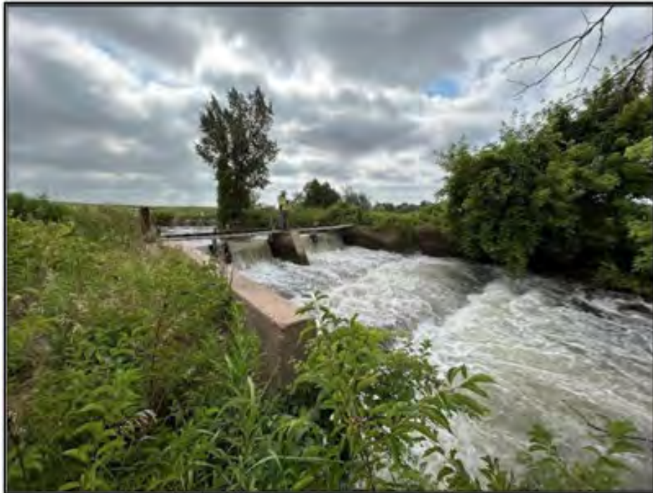
Figure 84. Birdwood Canal: Feature 1, diversion dam with crew member for scale. View to the southeast. Photograph taken on July 18, 2025.
