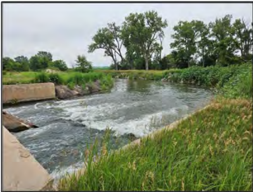
Figure 60. North Platte (Platte Valley) Canal, channel overview, Segment 1. View to the southwest below the headgate (Feature 1). Photograph taken on July 16, 2025.
