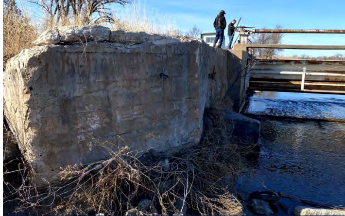
Figure 7. Retaining Wall at South Embankment – Downstream End
