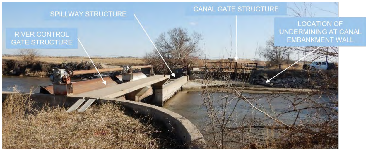
Figure 2. Looking South at Diversion structures.
