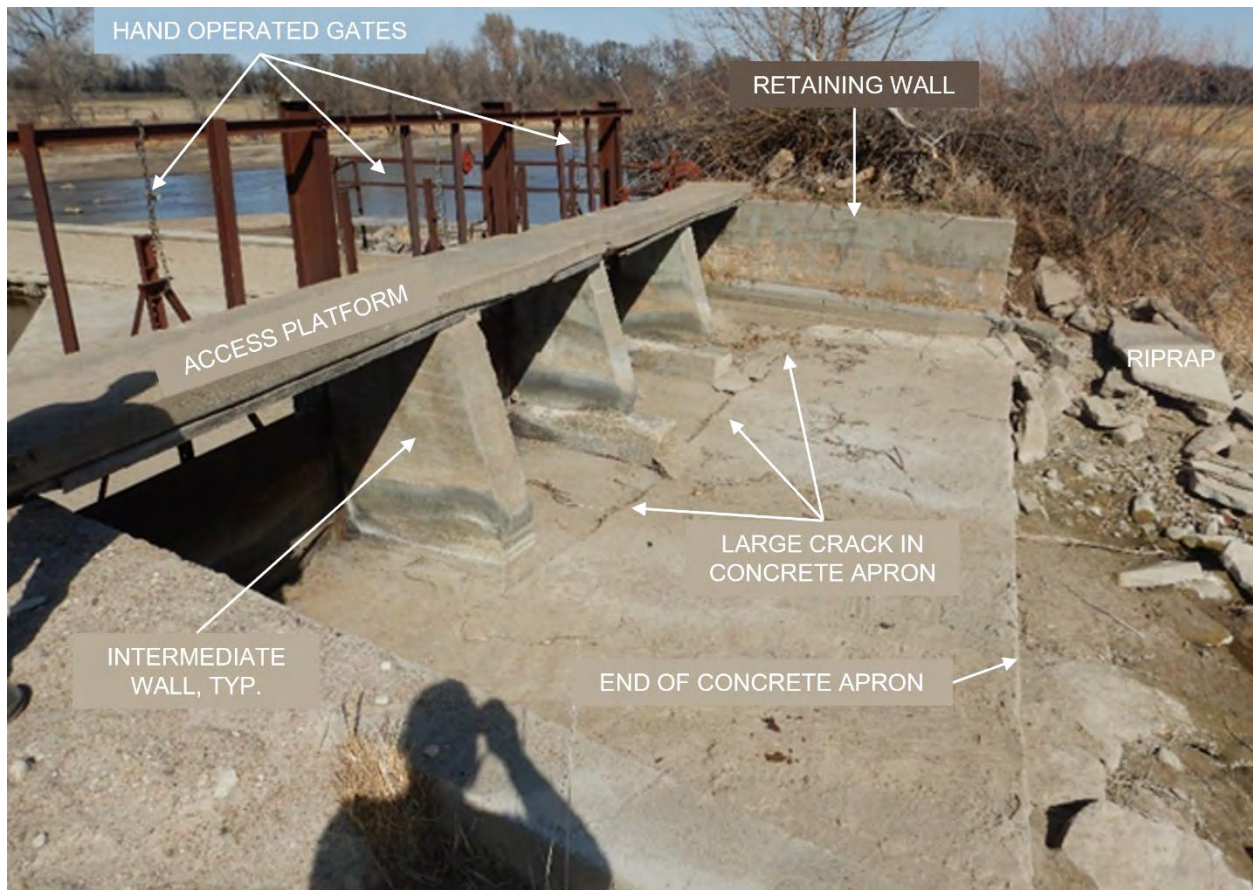
Figure 18. Looking Towards Canal Structure Outlet – Downstream End.
