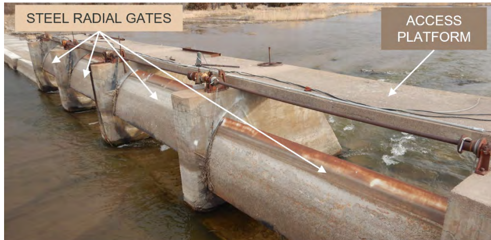
Figure 4. Looking North Towards River Gate Structure – Upstream End
