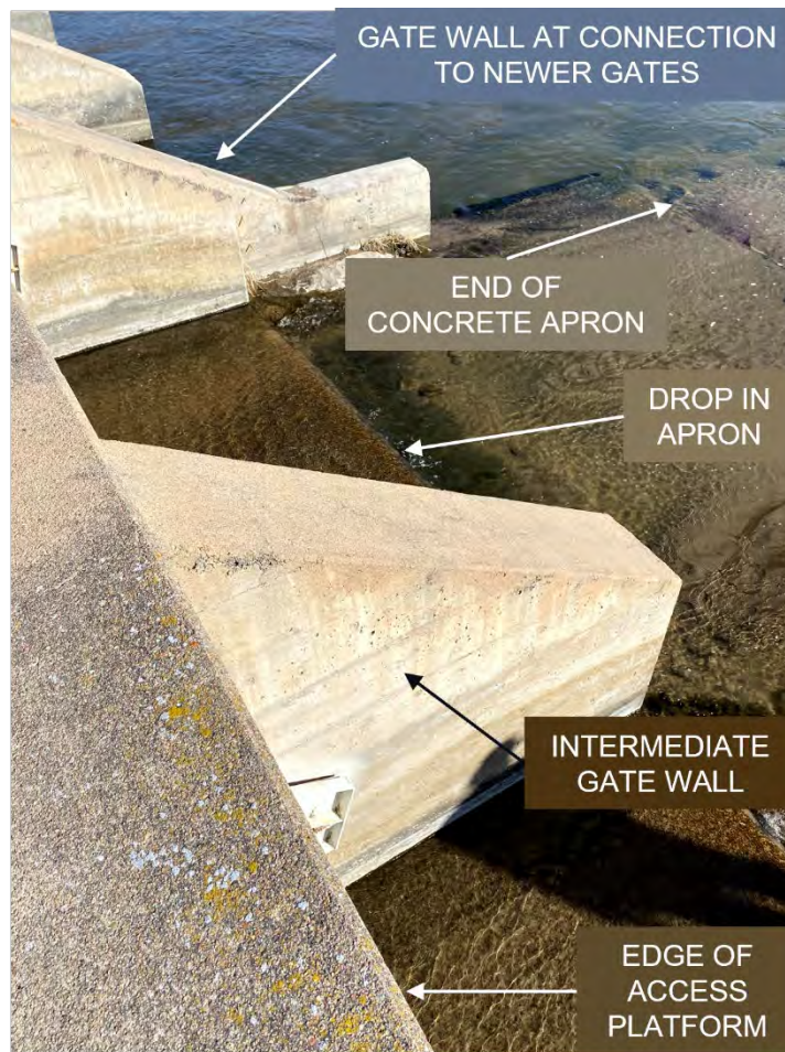
Figure 6. Walls of River Gate Structure – Downstream End
