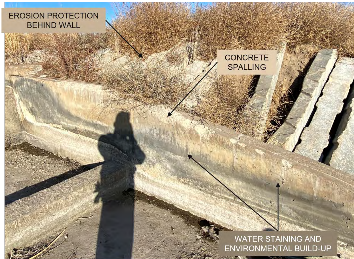
Figure 17. Retaining Wall at North Embankment – Downstream End
