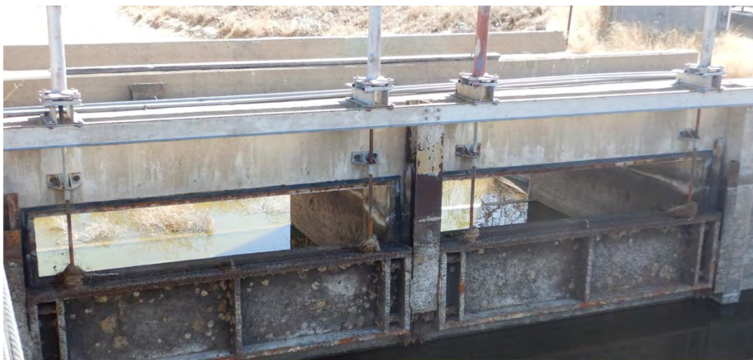
Figure 9. Looking Southeast Towards Canal Structure Inlet – Upstream End
