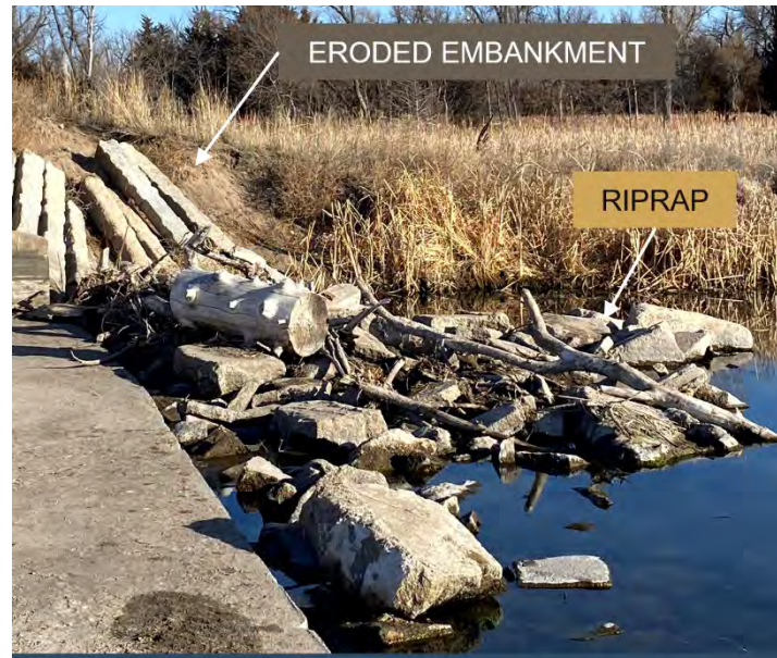
Figure 13. North Embankment – Downstream End
