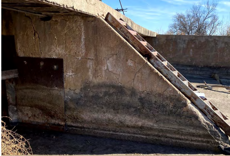
Figure 21. Intermediate Wall of Canal Gate Structure – Downstream End
