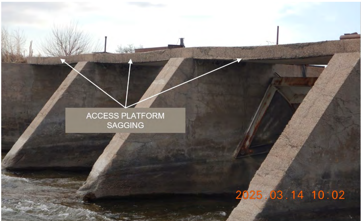
Figure 10. Typical Access Slab Sagging
