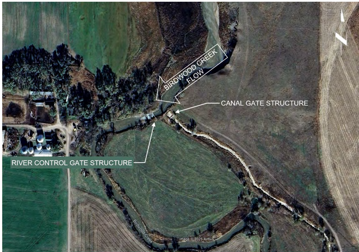
Figure 1. Site Map of Birdwood Irrigation District / Birdwood Creek Diversion Structure
