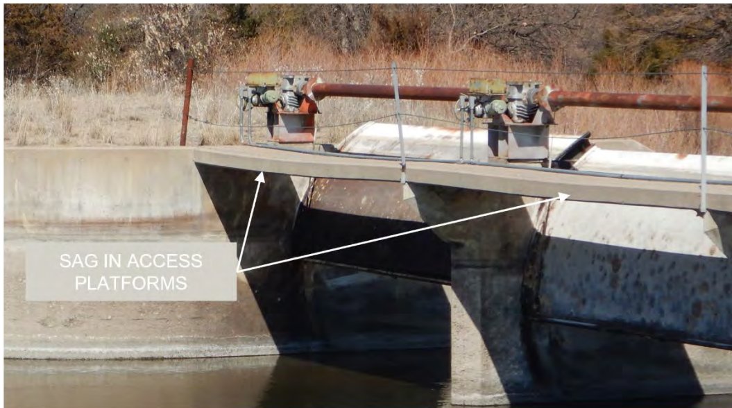
Figure 8. Typical Access Platform Condition
