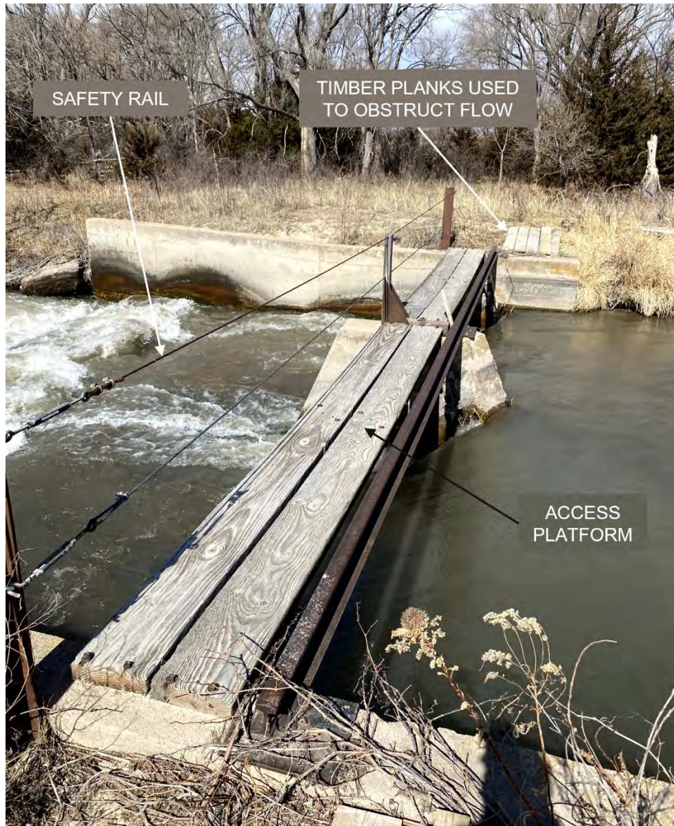
Figure 2. Looking Southeast Along River Control Gate Structure.
