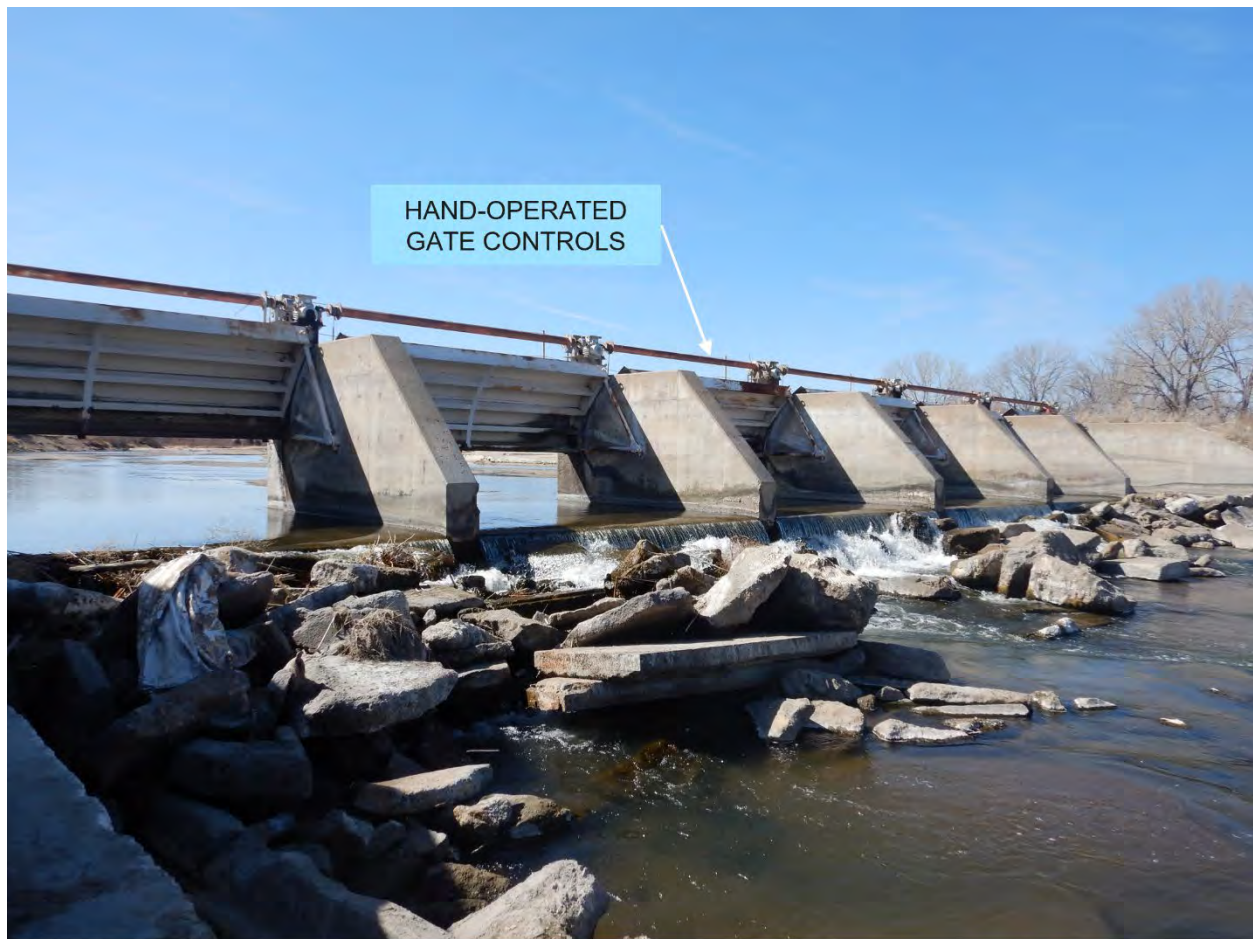
Figure 2. Looking Northwest Toward River Gate Structure – Downstream End
