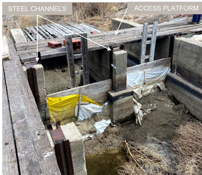
Figure 17. Looking East towards Canal Gate Structure – Upstream side
