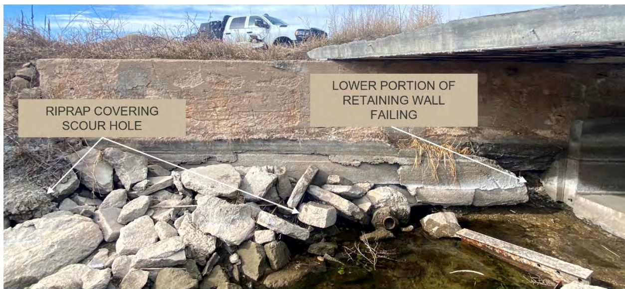
Figure 18. South Exterior Wall of Canal Gate Structure – Downstream End
