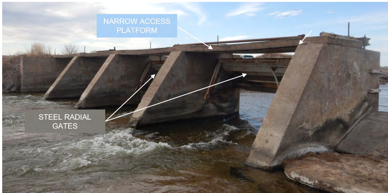
Figure 2. Looking South Toward River Gate Structure – Downstream End
