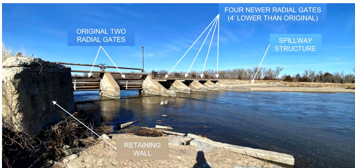
Figure 4. Looking Northwest Towards River Gate Structure – Downstream End
