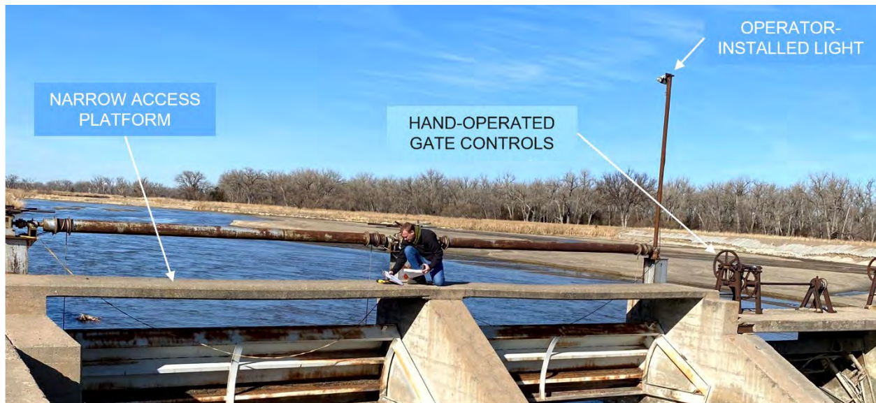
Figure 2. Looking Northwest Toward River Gate Structure – Downstream End
