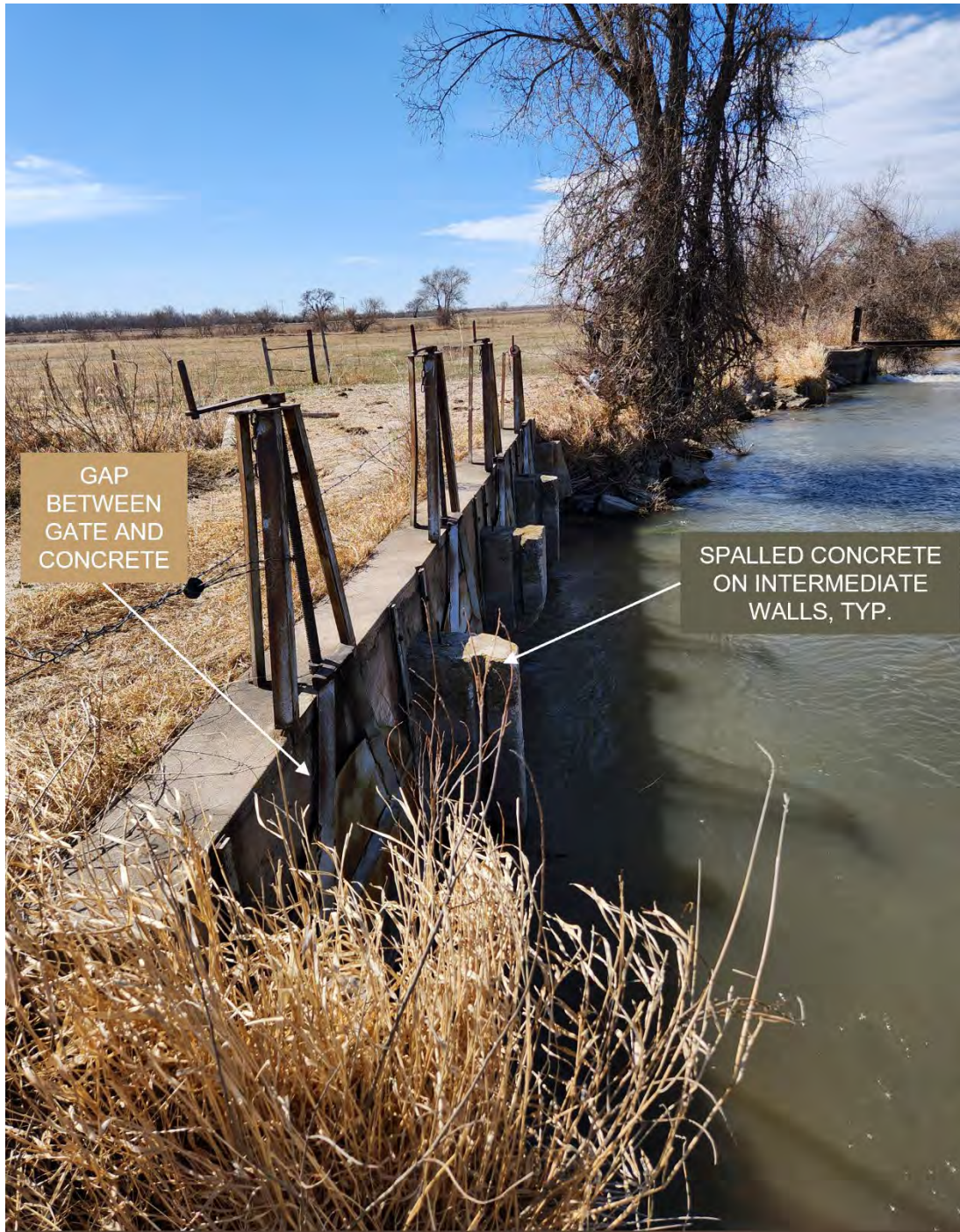
Figure 10. Inlet of Canal Gate Structure – Upstream side.
