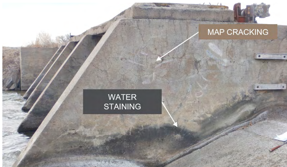
Figure 7. Typical River Gate Wall Condition
