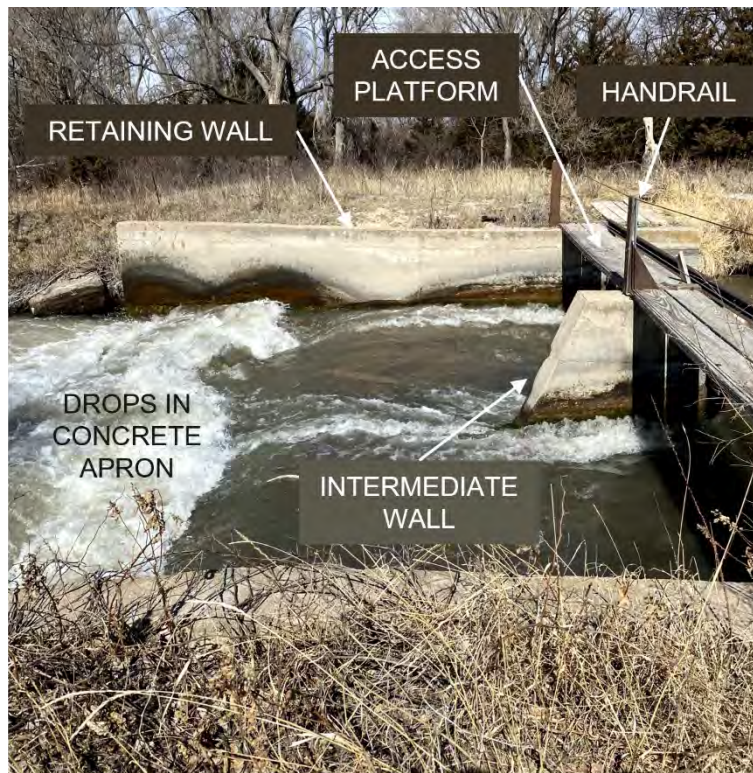
Figure 6. Looking South at River Control Gate Structure
