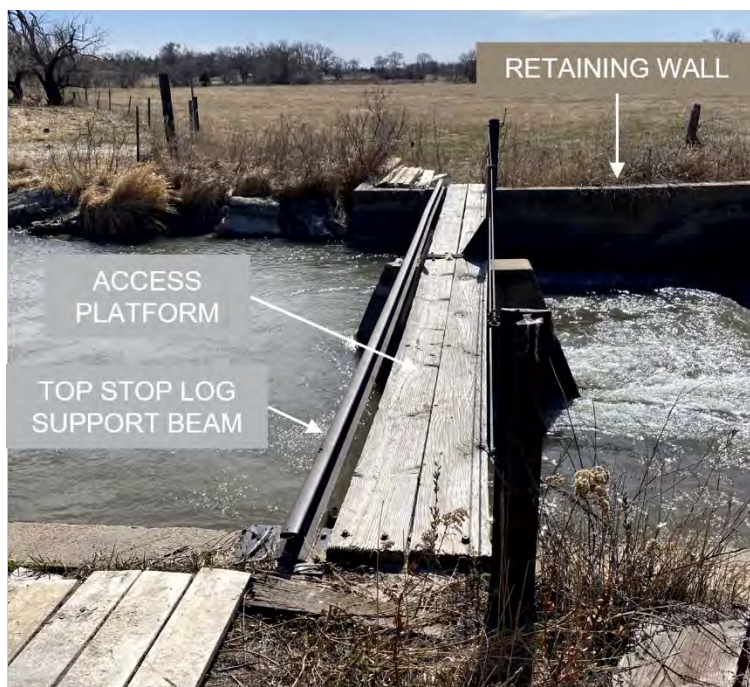
Figure 4. Looking Northwest Along River Control Gate Structure
