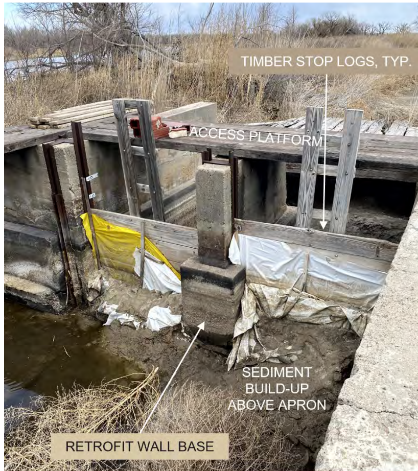
Figure 13. Canal Gate Structure Inlet – Upstream Side.
