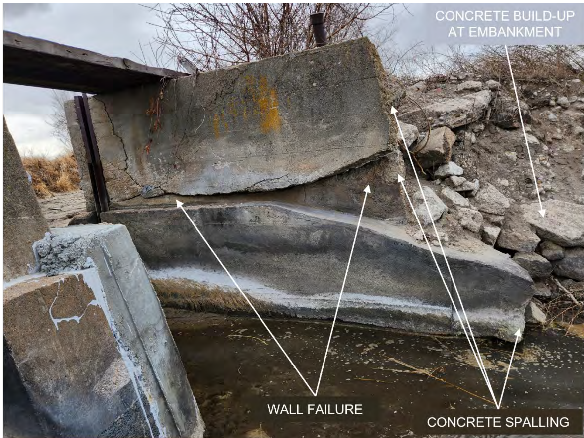
Figure 7. Southeast Retaining Wall at River Return Gate – Downstream side.
