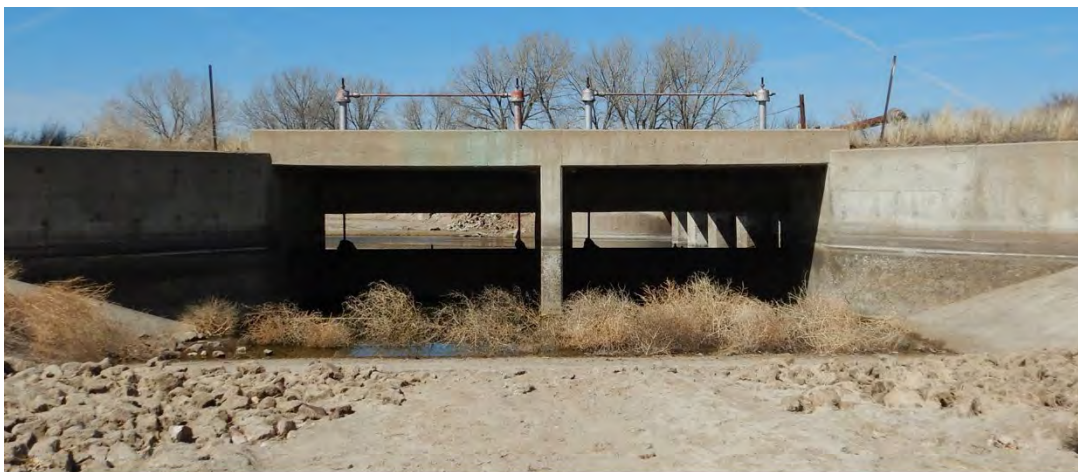
Figure 10. Looking Northwest Towards Canal Structure Outlet – Downstream End
