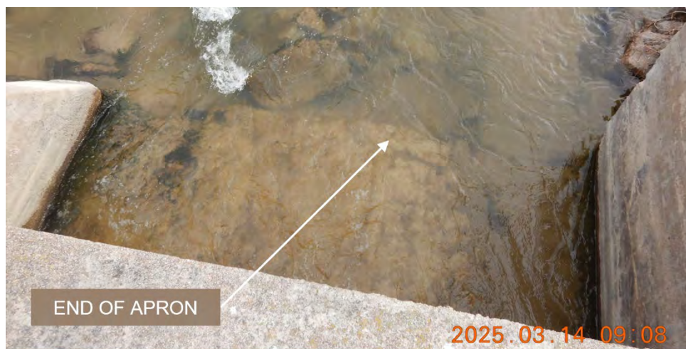
Figure 6. Concrete Apron and Drop off
