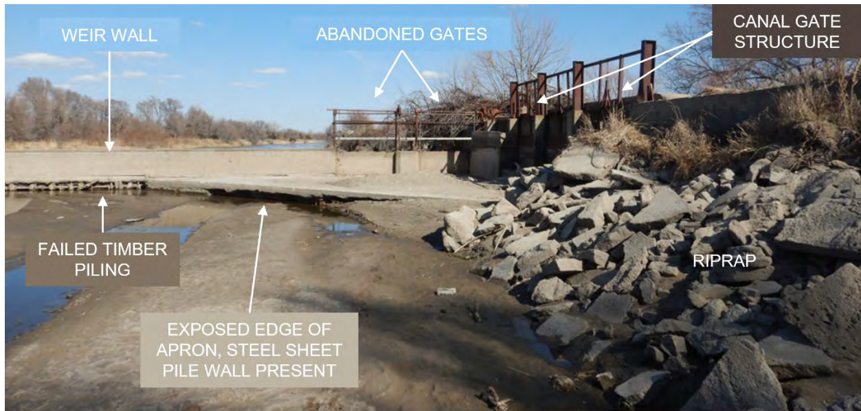
Figure 13. Spillway Structure and Canal Gate Structure – Upstream side.
