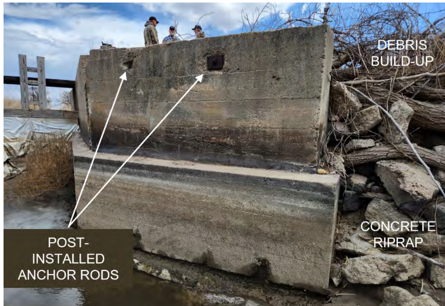
Figure 20. Southeast Retaining Wall of Canal Gate Structure.
