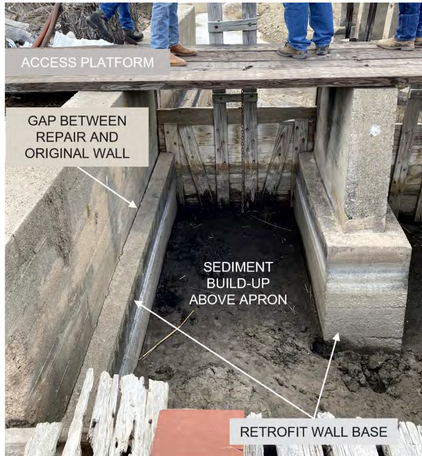
Figure 15. Looking at canal gates from downstream side.
