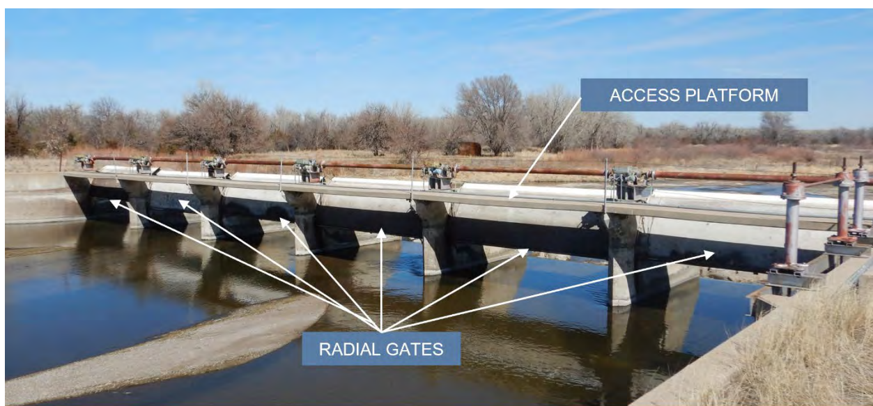
Figure 3. Looking Northeast Toward River Gate Structure – Upstream End
