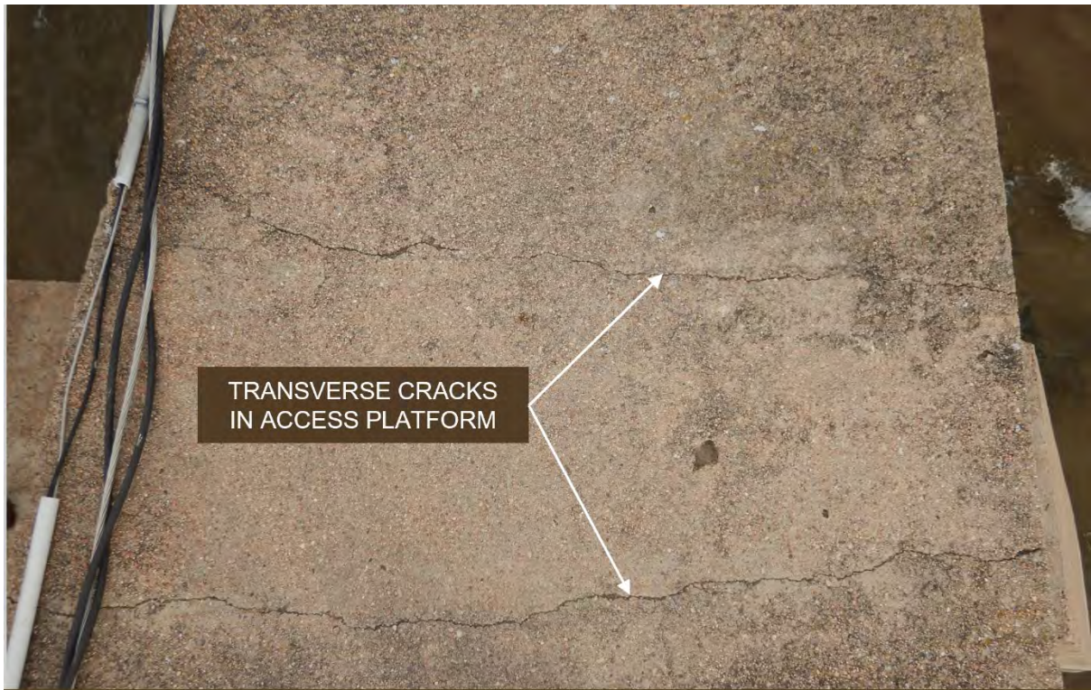
Figure 9. Typical Top of Access Platform Condition
