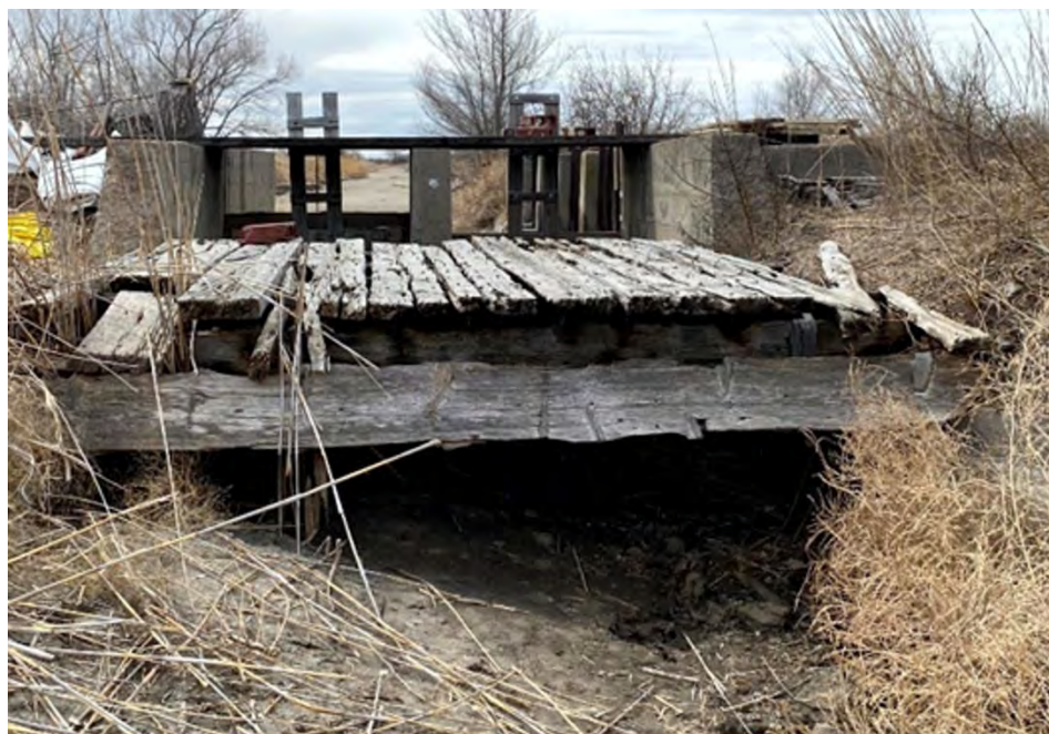
Figure 14. Retrofit Timber Access Bridge at Canal Gate Structure Outlet.
