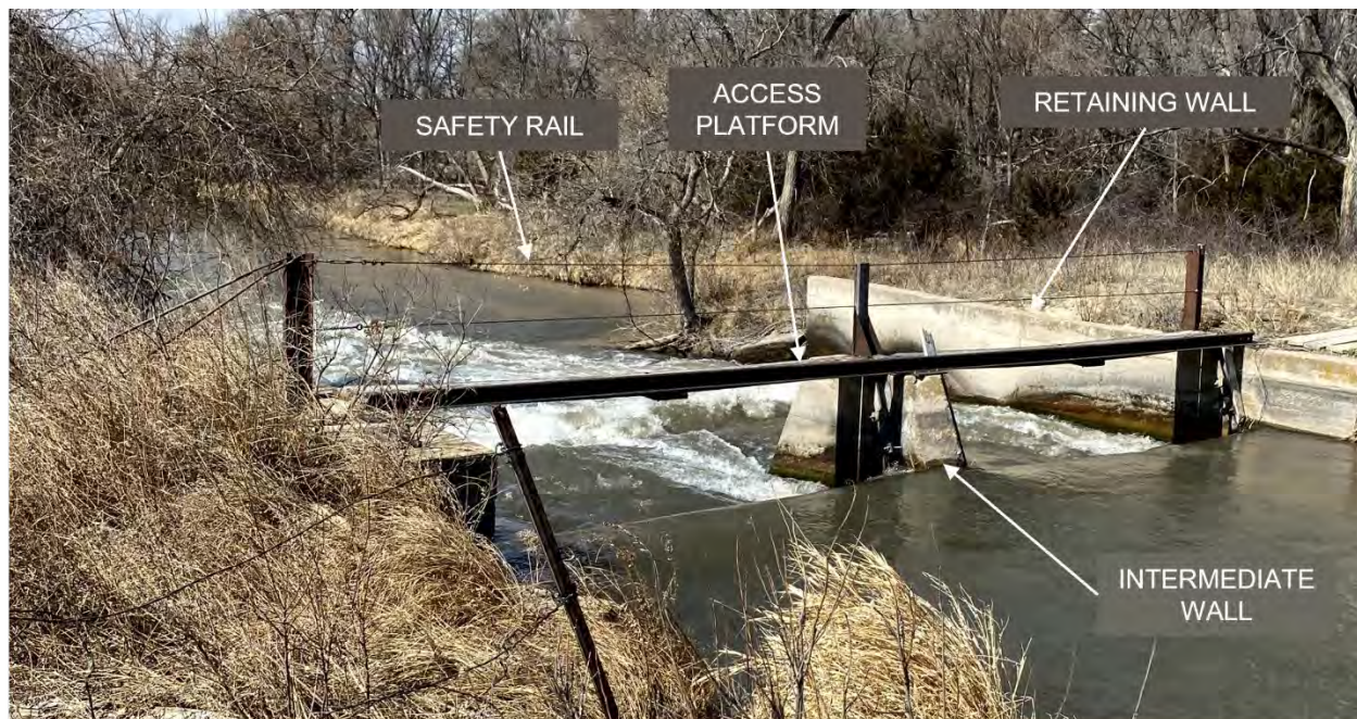
Figure 3. Looking Northeast Toward River Gate Structure – Upstream End
