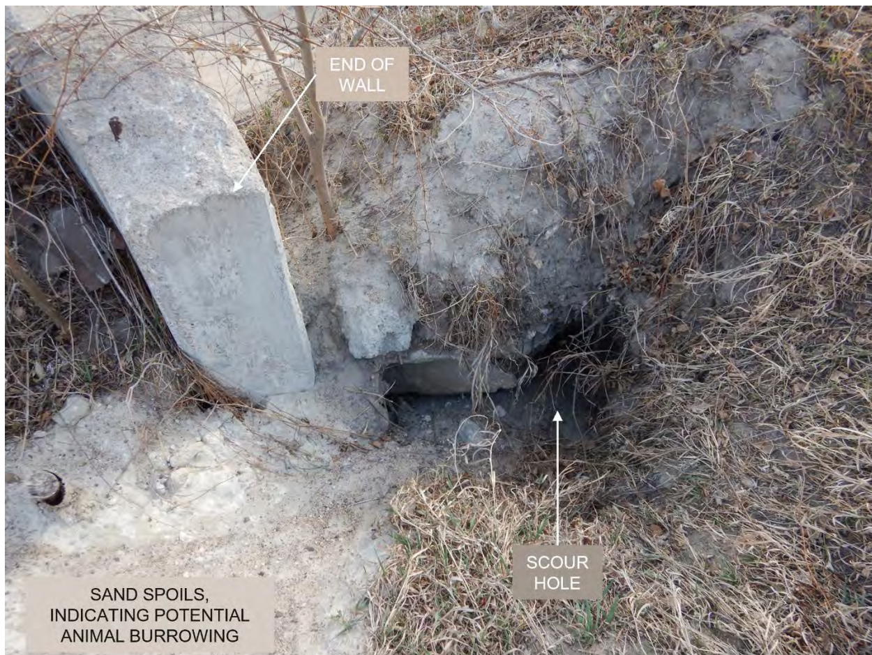
Figure 11. Upstream end of Northern River Control Gate Wall.
