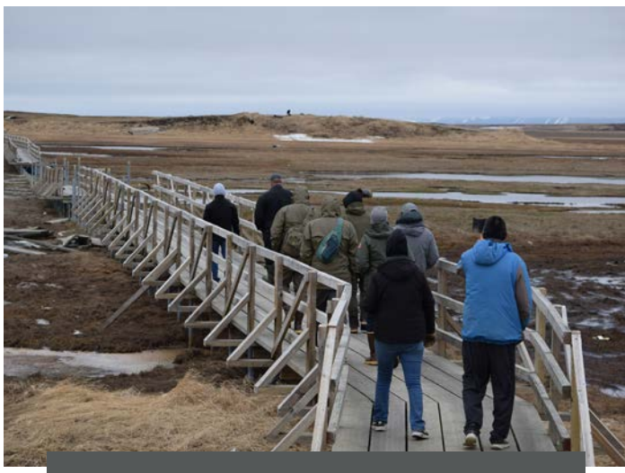
NRCS staff assess the rebuilding of the Hooper Bay Trail Project. The boarded walkway trail was damaged by Typhoon Merbok in 2022 and was rebuilt with EWP assistance. The project was completed in FY25. NRCS photo by Ann Fischer.
