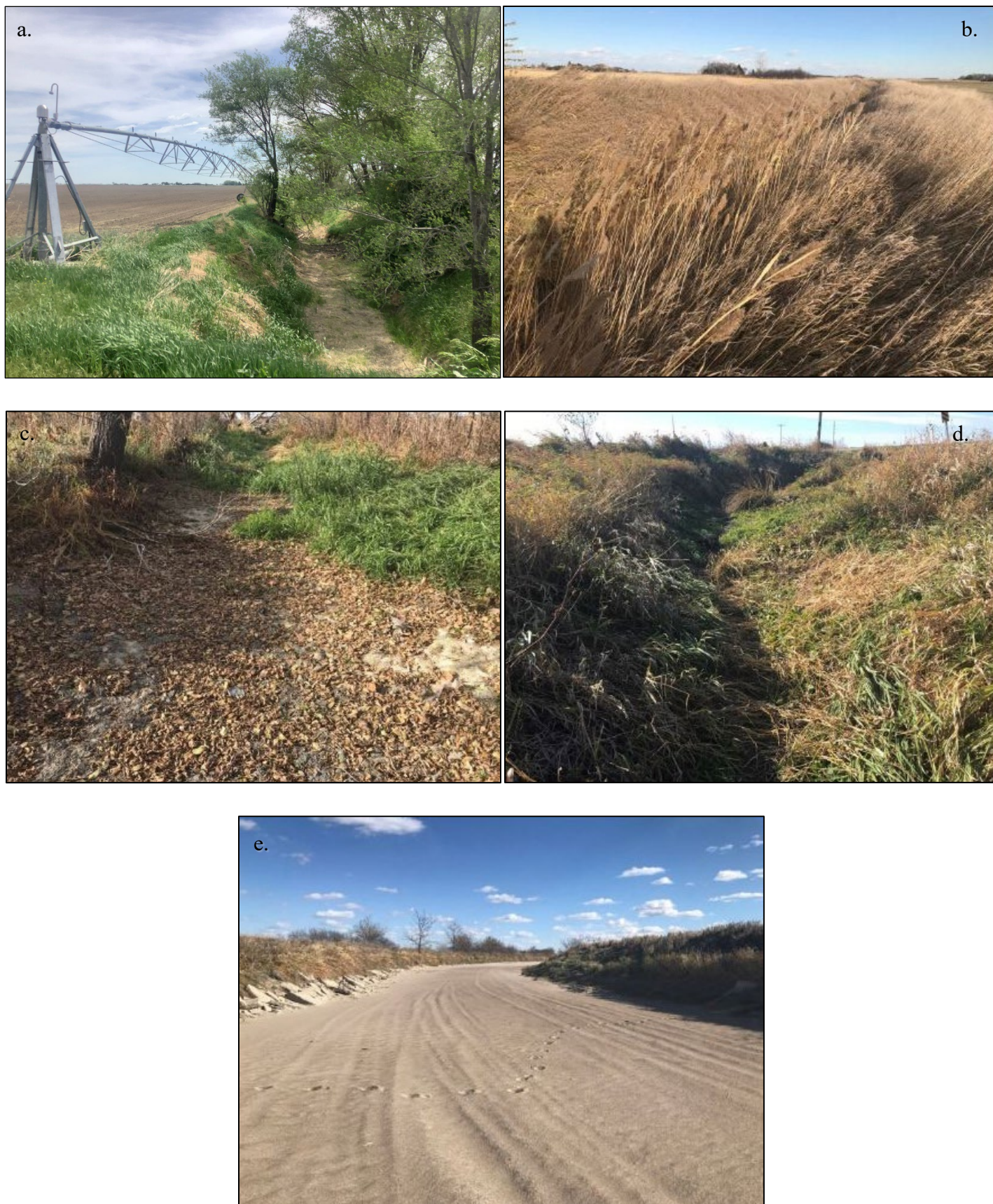
Figure 42. Examples of canal overgrowth, slumping, and shoring canal banks (a and b) north of Cozad, (c) east of Cozad along Country Club Road, (d) east of Cozad on Rd. 761, and (e) Dawson County Canal east of Cozad at northeast corner of Cozad Country Club, all within the Cozad APE.
