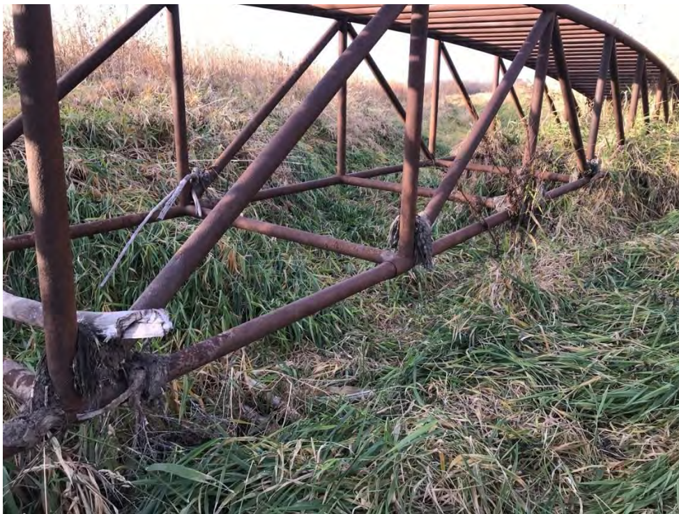
Photo 9 (W-13). Flow debris present on pivot bridge at W-13 indicating high flow events.
