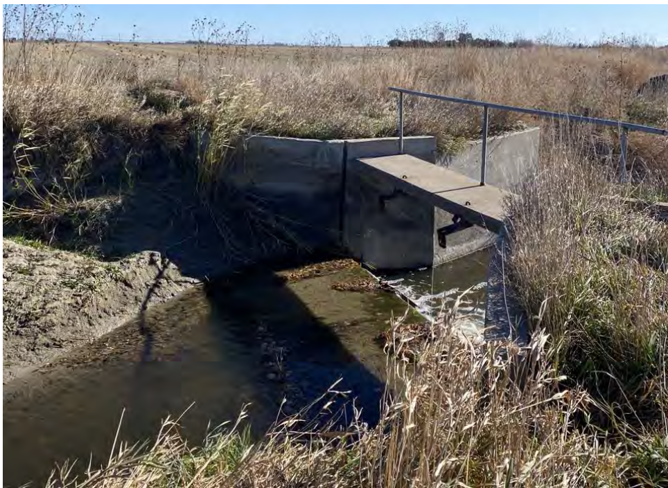
Photo 29 (S-6 and S-7). Headgate where streams S-6 and S-7 converge.
