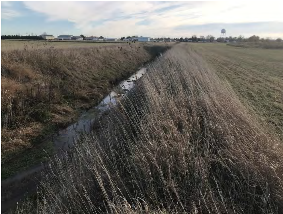
Photo 22 (S-2) . Stream S-2 facing south. Note the height of banks due to the berms built on the sides of the stream.
