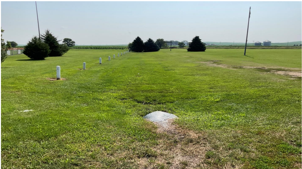
Photo 18 – View looking east from 4 th Street. Photo depicts a culvert structure within the roadside ditch. No wetlands were present.
