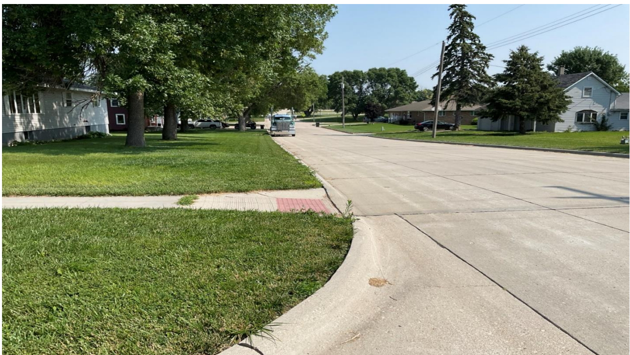
Photo 22 – View looking north along the west side of N Hill Street. Photo depicts mowed upland vegetation within the roadside ditch.
