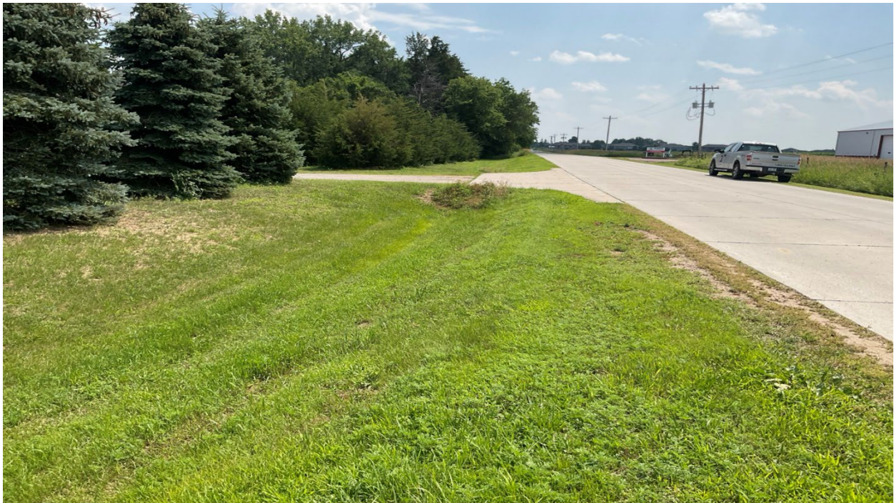
Photo 61 – View looking south along the east side of 549 th Avenue. Photo depicts an upland roadside ditch.
