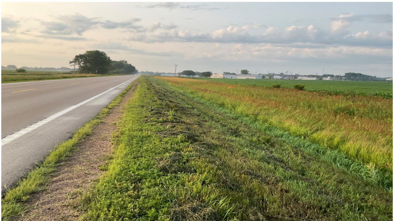
Photo 72 – View looking southeast along the south side of Highway 13. Photo depicts an upland roadside ditch.
