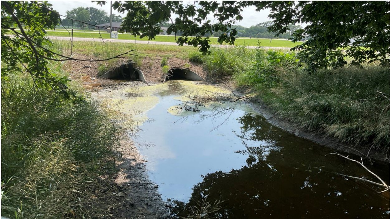
Photo 113 – View looking southwest along Unnamed Stream 7. Photo depicts the OHWM of the stream and PEM Wetland KK.
