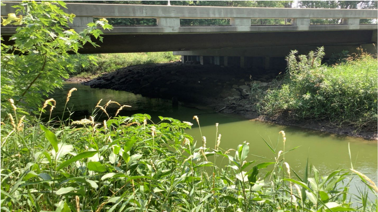
Photo 205 – View looking northeast on the west side of Highway 13. Photo depicts PEM Wetland TTT along Willow Creek.
