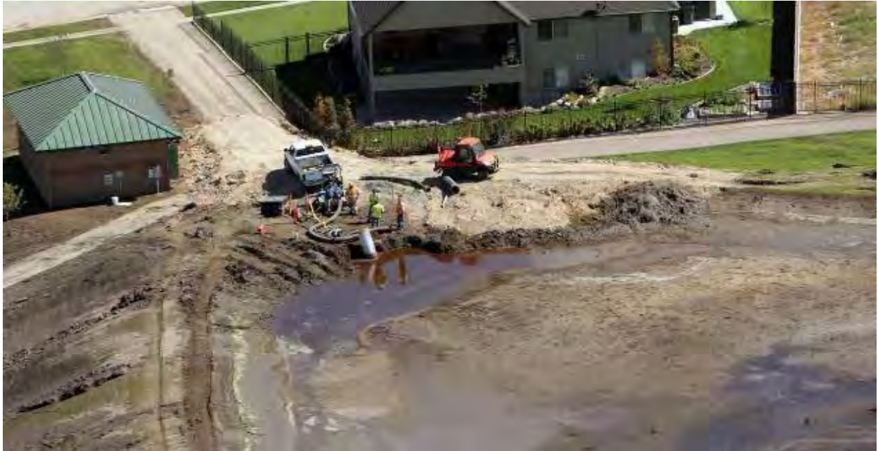
Photo 2. Sedimentation and flood damage from September 4, 2012
