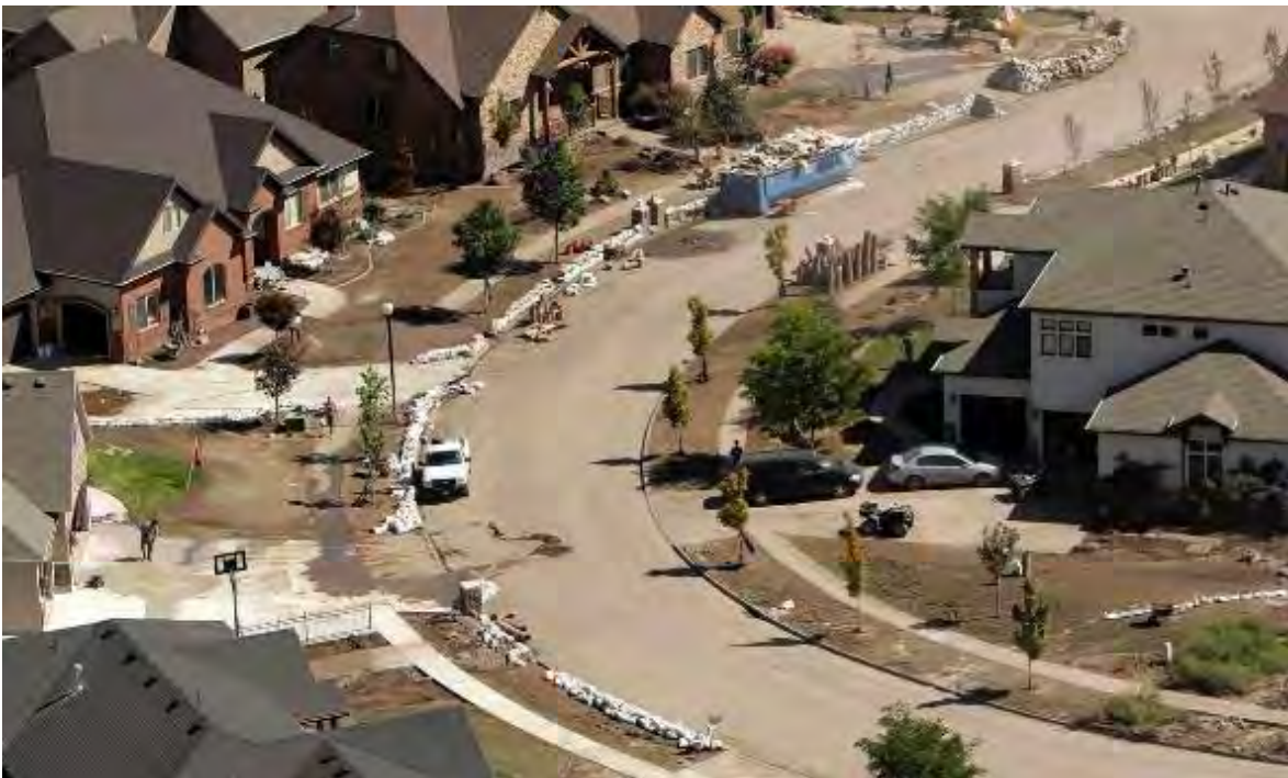
Photo 7. Sedimentation and flood damage from September 4, 2012
