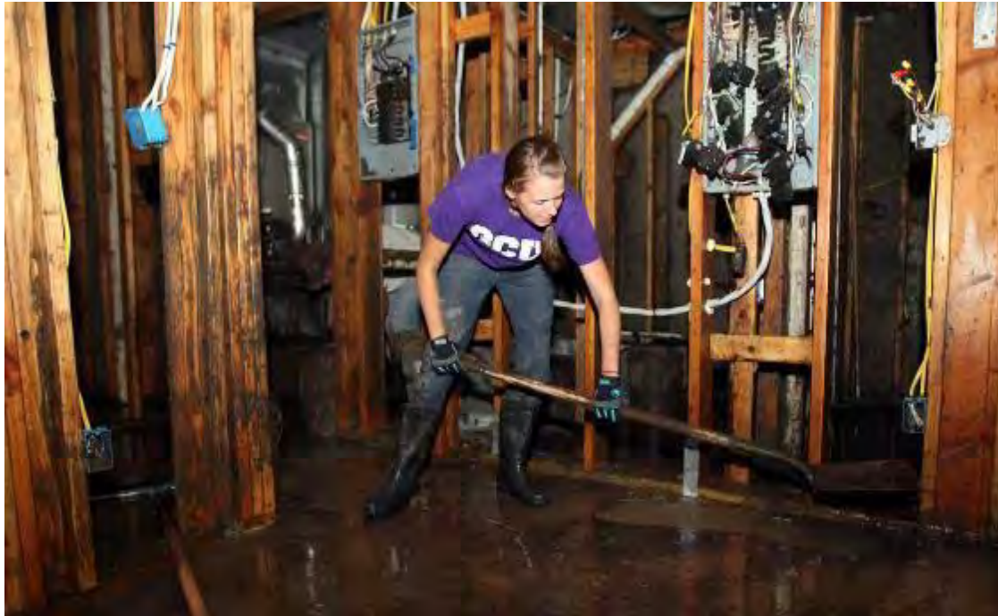
Photo 4. Basement flood damage from September 4, 2012
