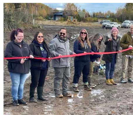
Representatives from the Native Village of Tyonek and the Tyonek Tribal Conservation District, with other agency partners, at a ribbon cutting ceremony for a culvert fish passage project in Tyonek, Alaska.
