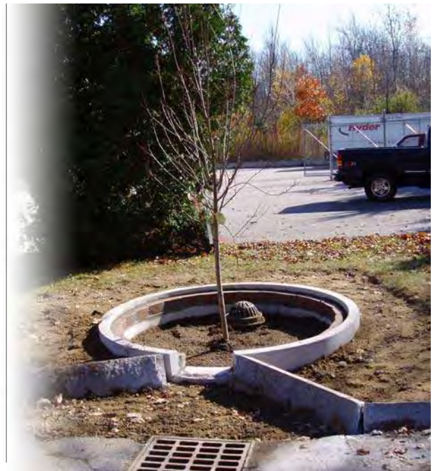
Example tree box filter design (UNH Stormwater Center 2007a) and installation in the Hodgson Brook Watershed in Portsmouth, NH.
