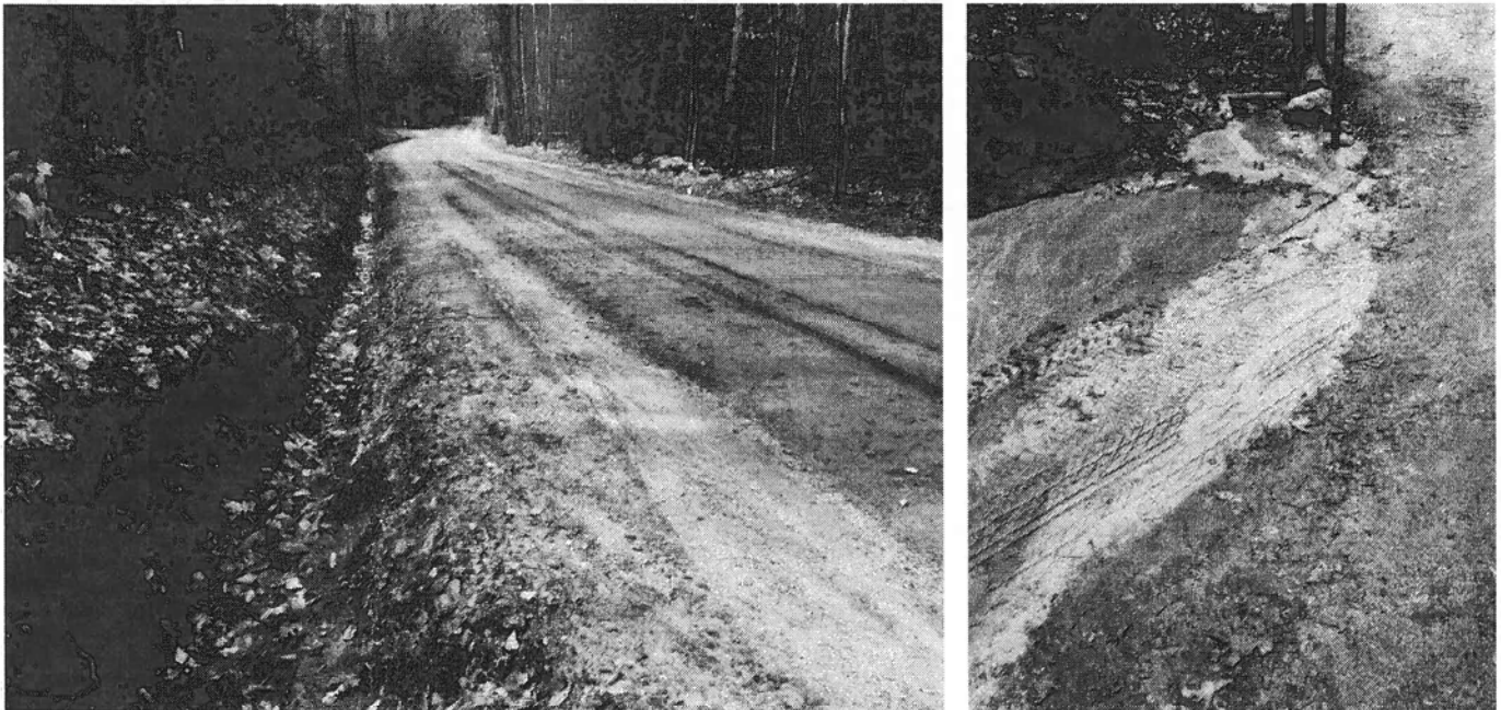
Figure 8. (Left) View of the roadside ditch erosion present along Kaulback Road far north. (Right) Erosion at the base of the steep driveways.
