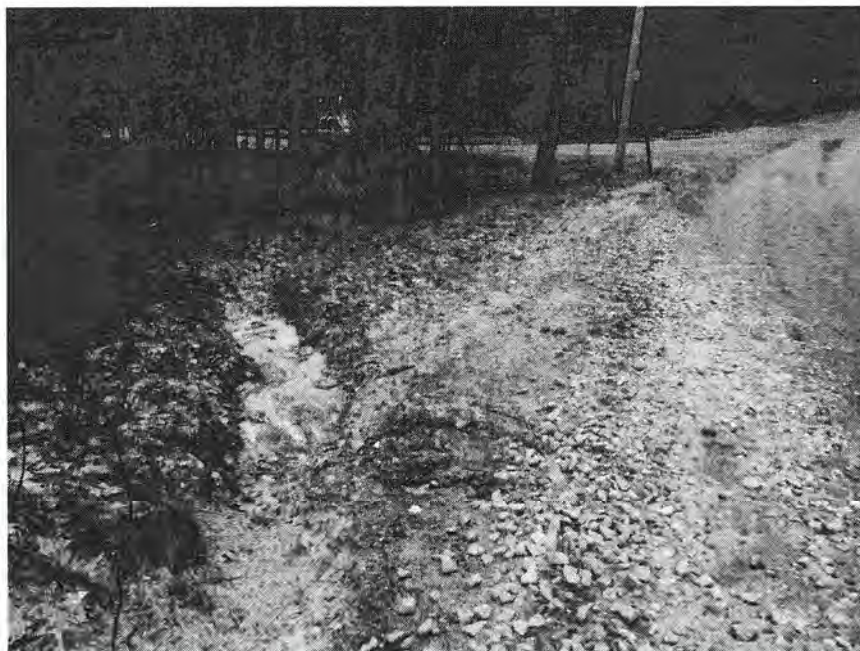
Figure 13. View of eroding turnout on Roxbury Road.
