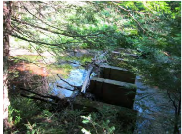
Photo 4- Stop Log Dam Closer
