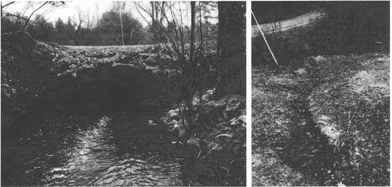
Figure 11. (Left) View of Woodman Road-unnamed stream crossing outlet. (Right) Eroded channel at the outlet of small culvert under the Union Cemetery Road.
