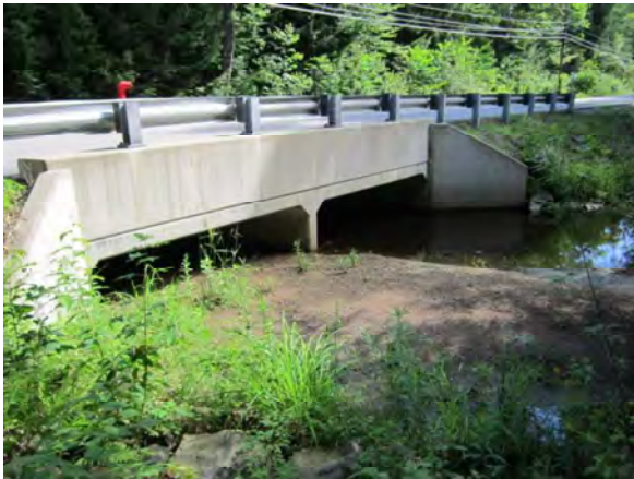
Photo 1 – Upstream Box Culverts
