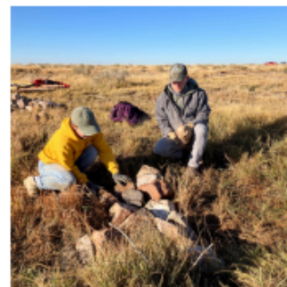
Emma Califf building a Zeedyk structure at a restoration workshop. Photo: Patty Knupp
