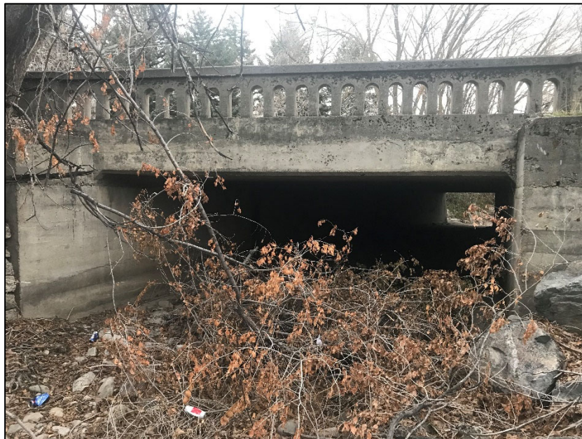
Photo 4. 300 North Upstream of Box Culvert.
