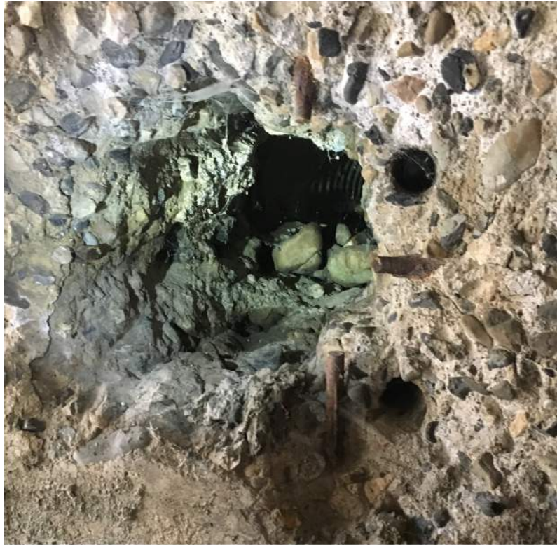
Photo: Storm Drain in Side of 200 South Culvert
