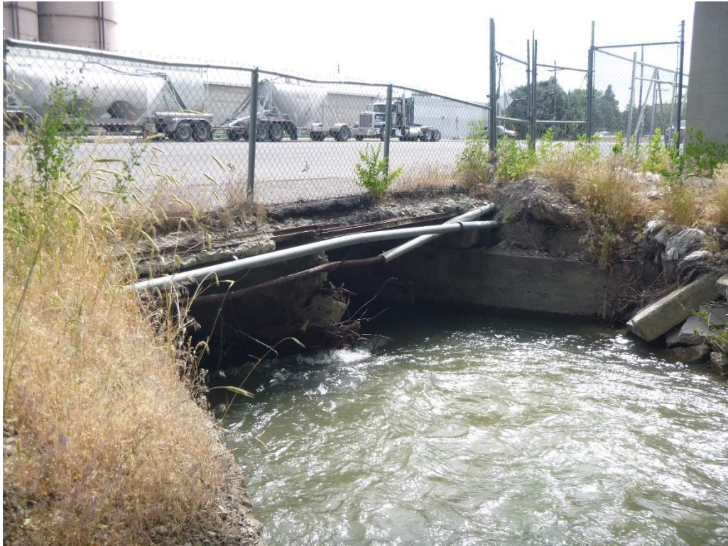
Photo 1. Upstream condition of box culvert at 100 North and 200 East (Location 5).
