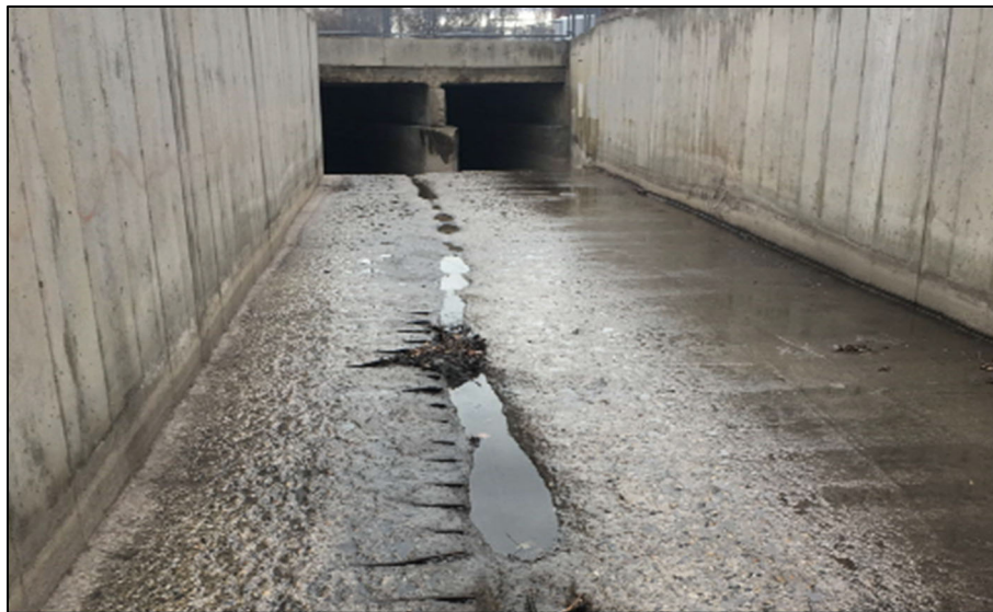
Photo 12. Open Channel Groove in Floor.
