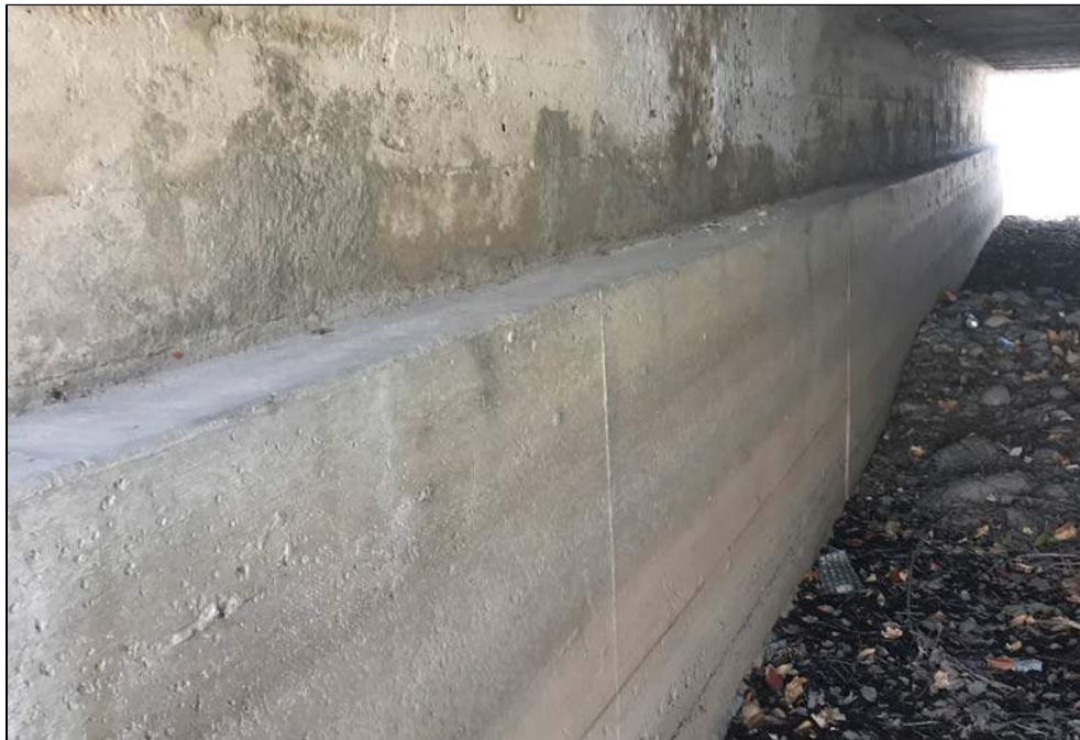
Photo: 200 South Culvert Recent Repair
