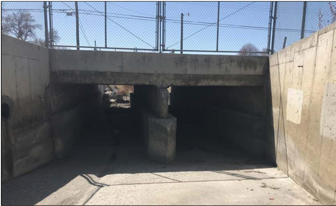
Photo: 200 South Box Culverts
