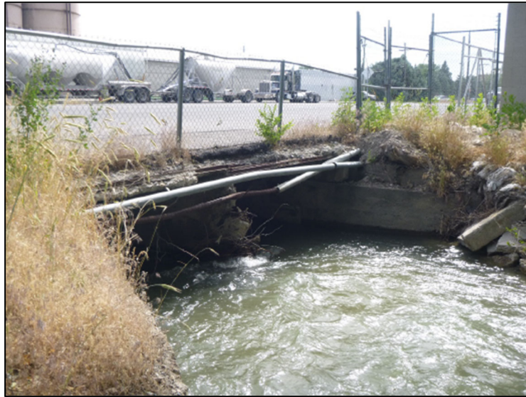
Photo 7. Upstream Condition of Box Culvert.
