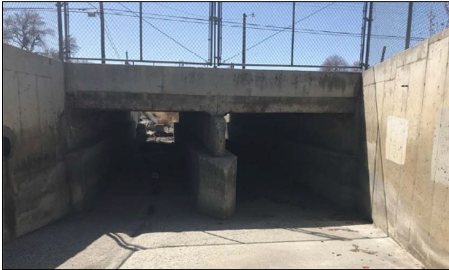
Photo 13. 200 South Box Culverts.
