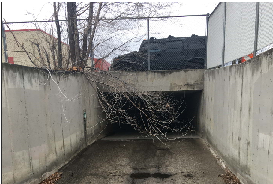
Photo: Exit of Box Culvert
