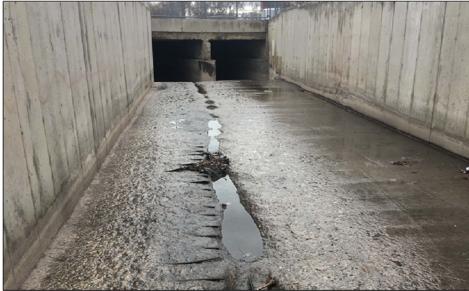
Photo: Open Channel Groove in Floor
