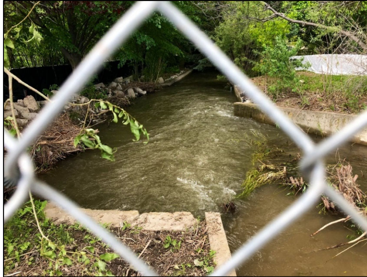
Photo 22. Dry Creek Channel at Capacity. Photo Credit Matt Rascon.
