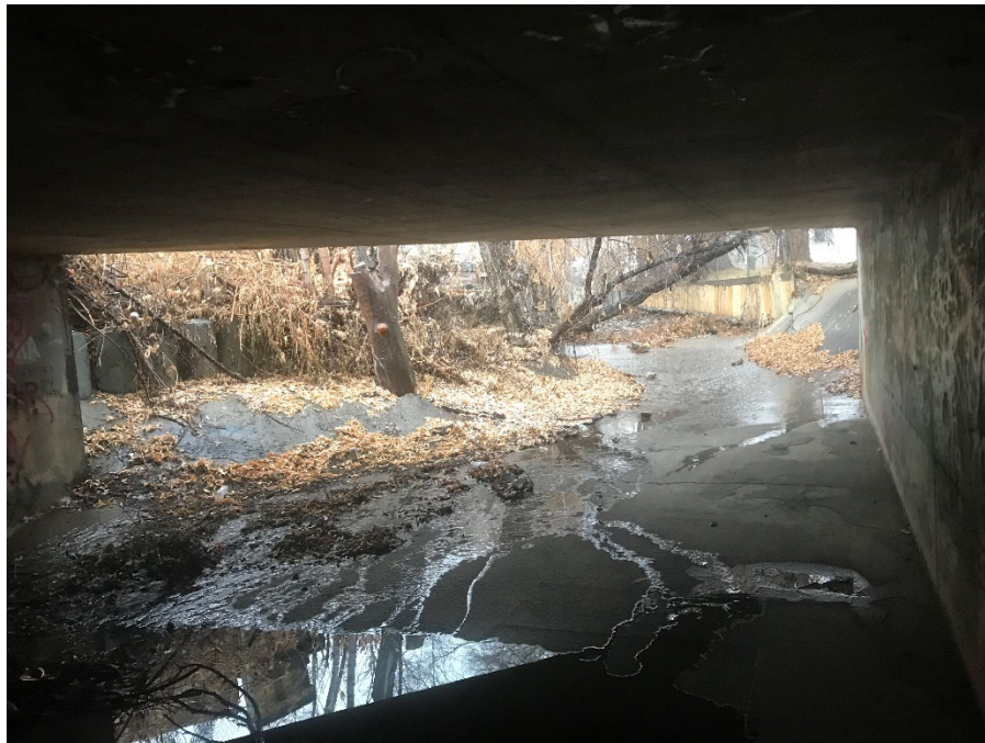
Photo 17. Transition into 400 South Box Culvert.
