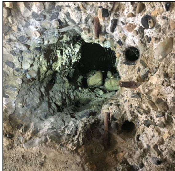
Photo 15. Storm Drain inside of 200 South Culvert.
