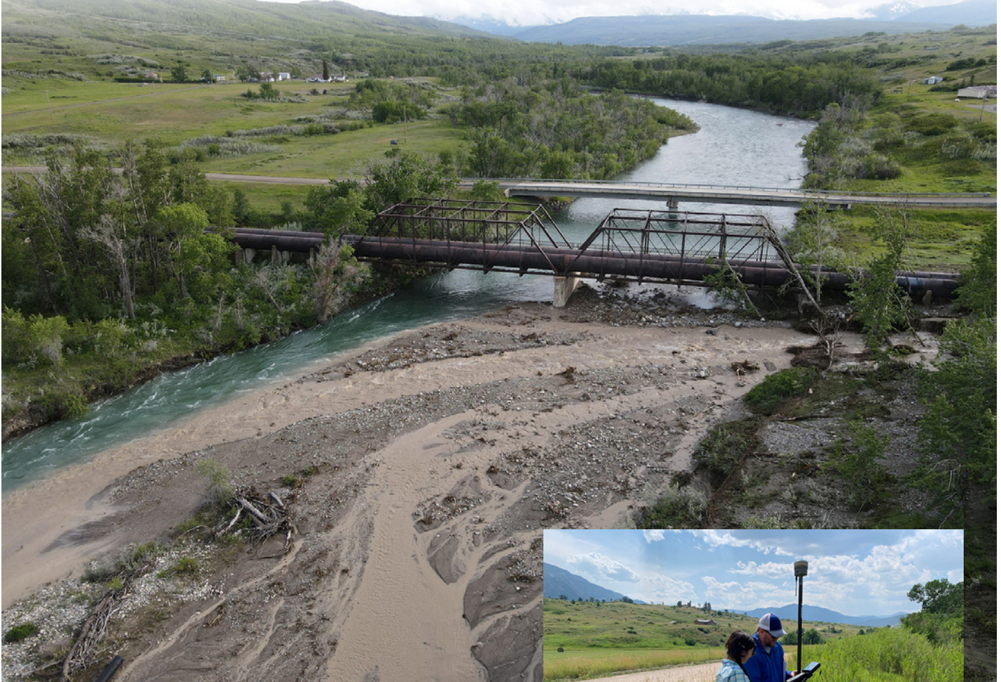
Sediment washed into the St. Mary River when the siphon structures failed in 2023. Photo courtesy Milk River Project.
