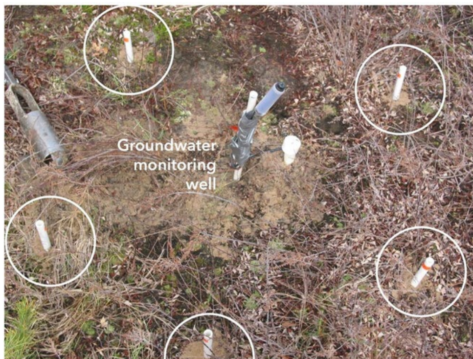
Figure 4.—Equipment installed in support of HSTS data collection. Note that a nest of five IRIS devices (circled) surround a shallow groundwater table monitoring well. The well is outfitted with an automated data logger (Berkowitz et al., 2021).
