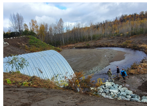
Tyonek TCD is working with many partners including USDA to install fish passage culverts to improve salmon habitat.
