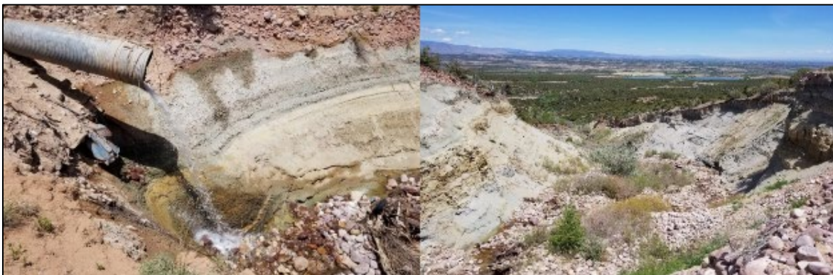
Figure 2-2: Coyote Canal Erosion
