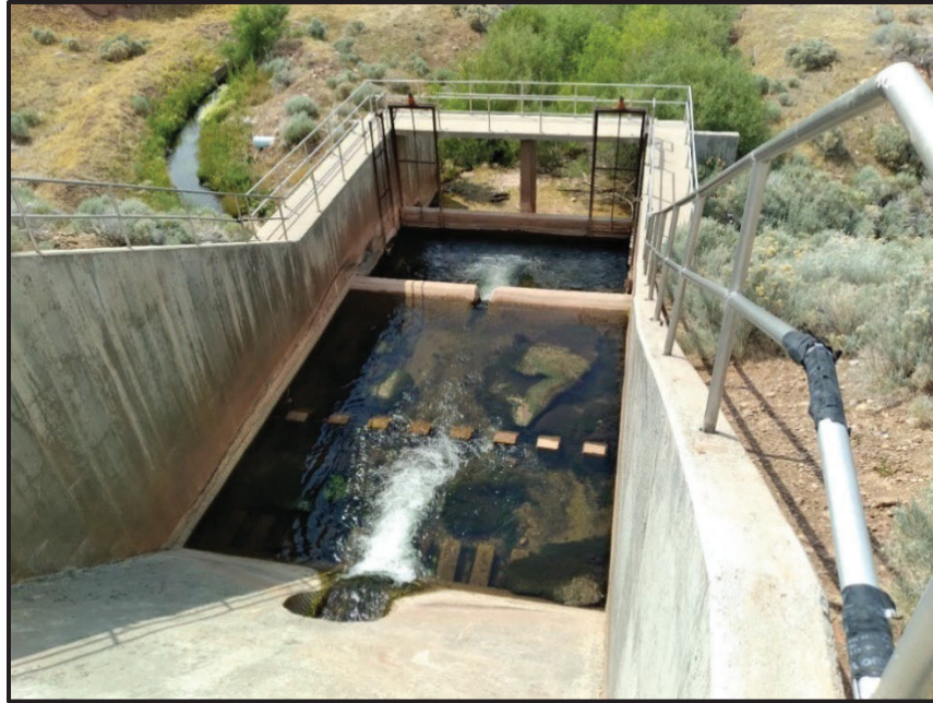
Figure 2: Outlet Works Stilling Basin, June 2021
