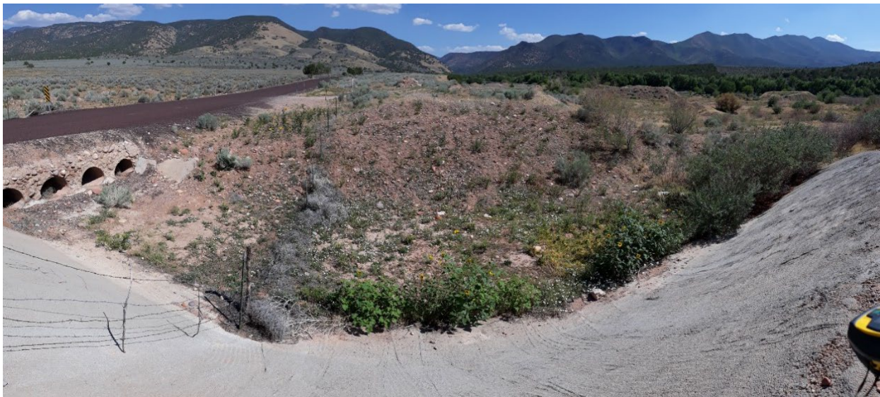
Figure 3-9: Emergency Spillway Culverts Upstream End
