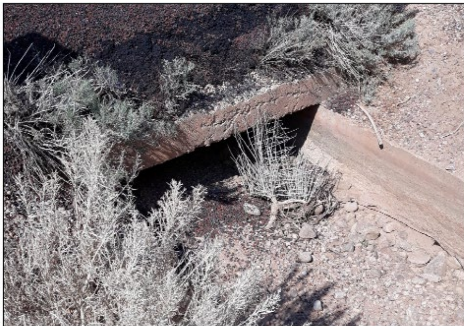
Figure 3-19: Box Culvert under Highway 106 for the East Field Single Ditch
