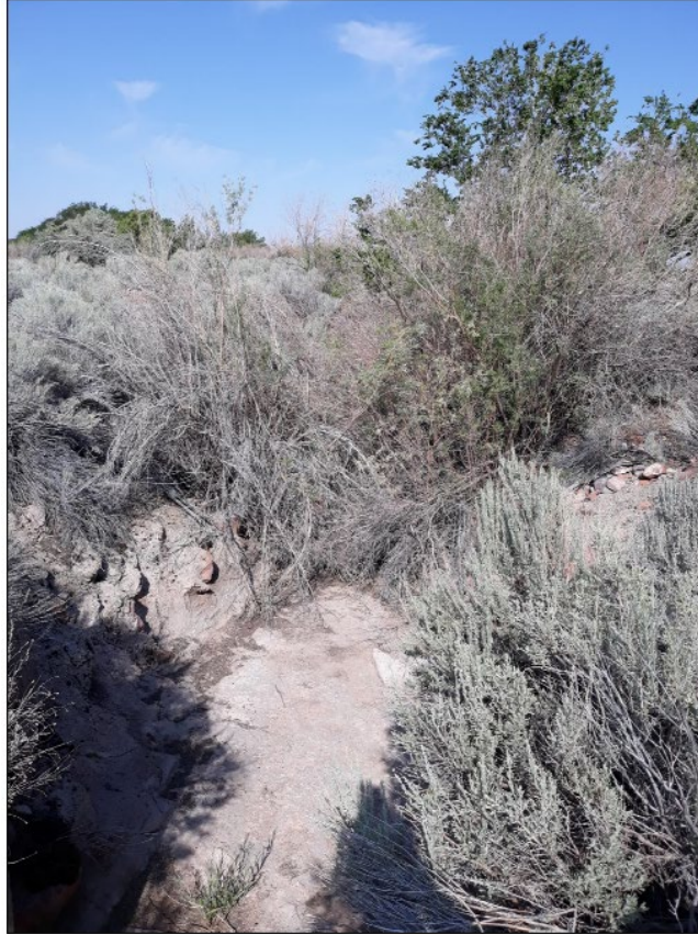
Figure 3-18: South Single Ditch Just Downstream of the Diversion Structure
