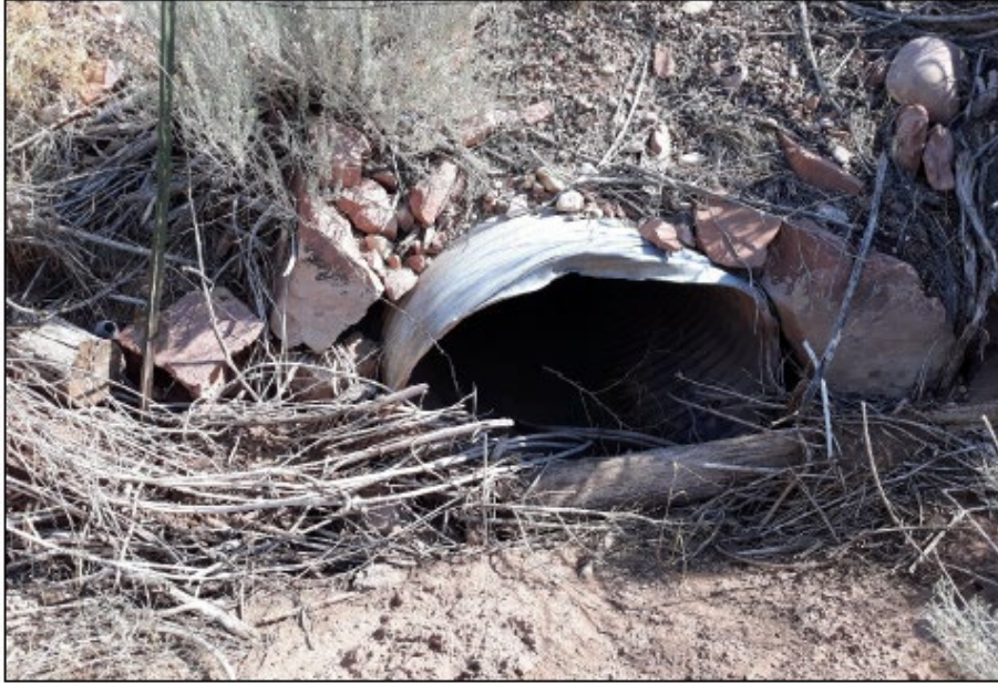
Figure 3-14: One of the Culverts Crossing Highway 106 for the East Field Single Ditch
