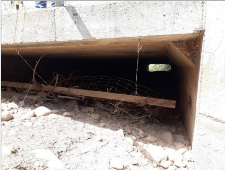
Figure 3-15: Box Culvert Crossing at Highway 133
