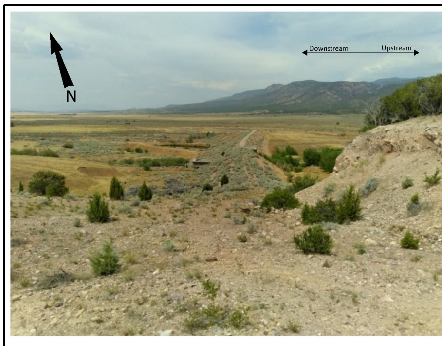
Figure 3-2: Dam Embankment – West End View
