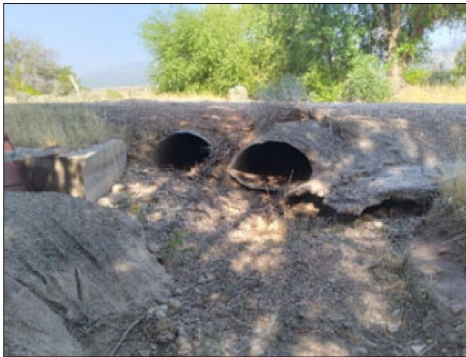
Figure 3-17: Double Culvert on South Single Ditch
