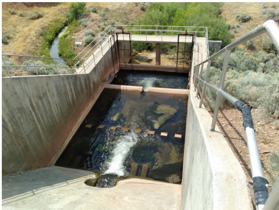
Figure 3-7: Primary and Secondary Spillway Stilling Basin
