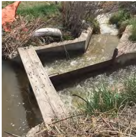
Figure 47. Proportional splitter at the bifurcation of the Jesse Lateral
