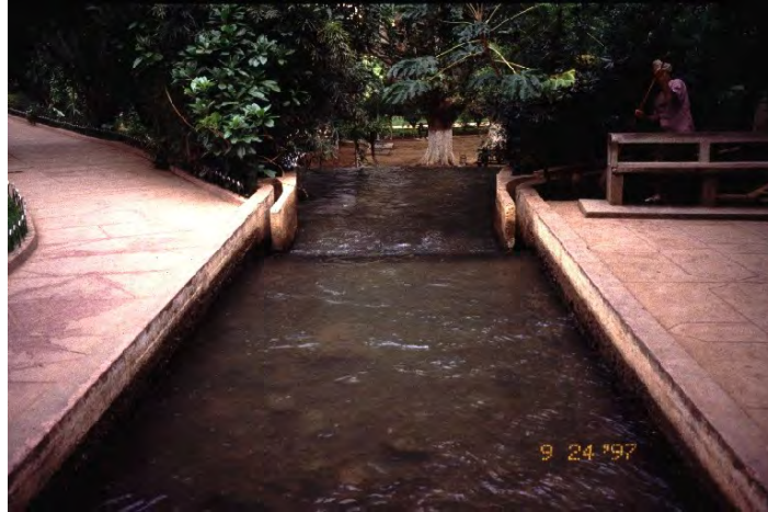
Figure 77. Proportional distributor near Beni Amir, Morocco. One large flow is split into two smaller flows (one on each side), and one big flow in the middle.
