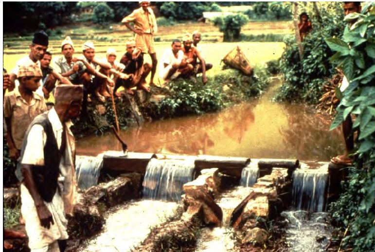
Figure 76. A simple but effective proportional control structure to equitably divide a stream flow in which the flow rate constantly varies.
