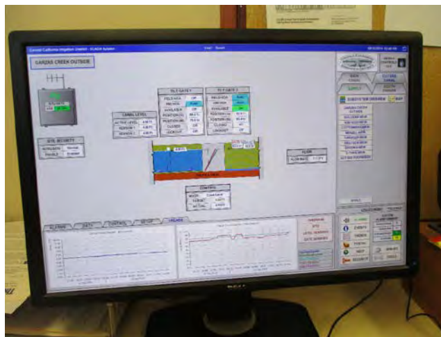
Figure 83. Relatively advanced HMI screens at Central California Irrigation District with numerical displays, control capabilities and trend lines
