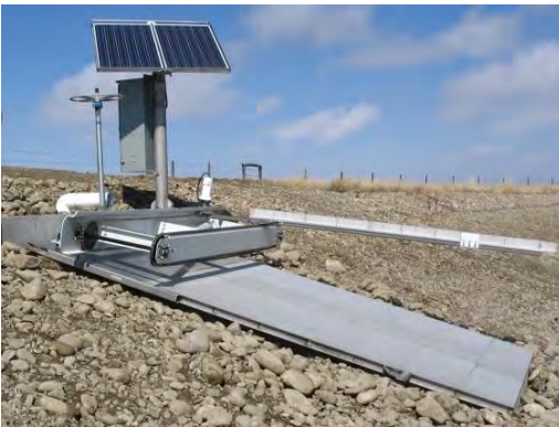
Figure 54. Self-sweeping screen and trash rack cleaner manufactured by Aqua Systems 2000 Inc.
