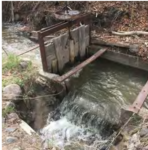
Figure 45. Flow control gate to set the target flow rate into the Jesse Lateral
