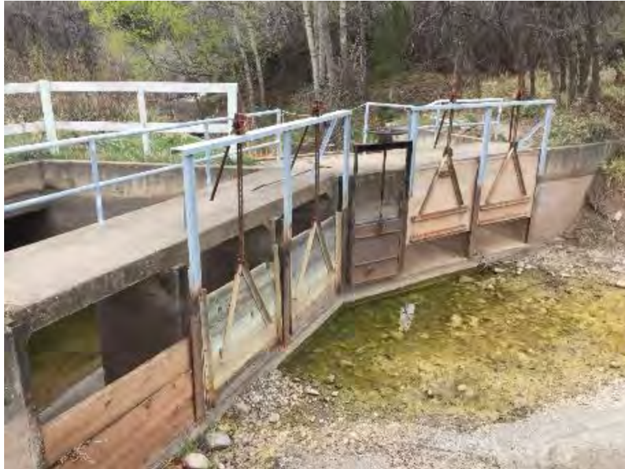
Figure 17. Terror Creek structure. The right hand two sluice gates control the spill.
