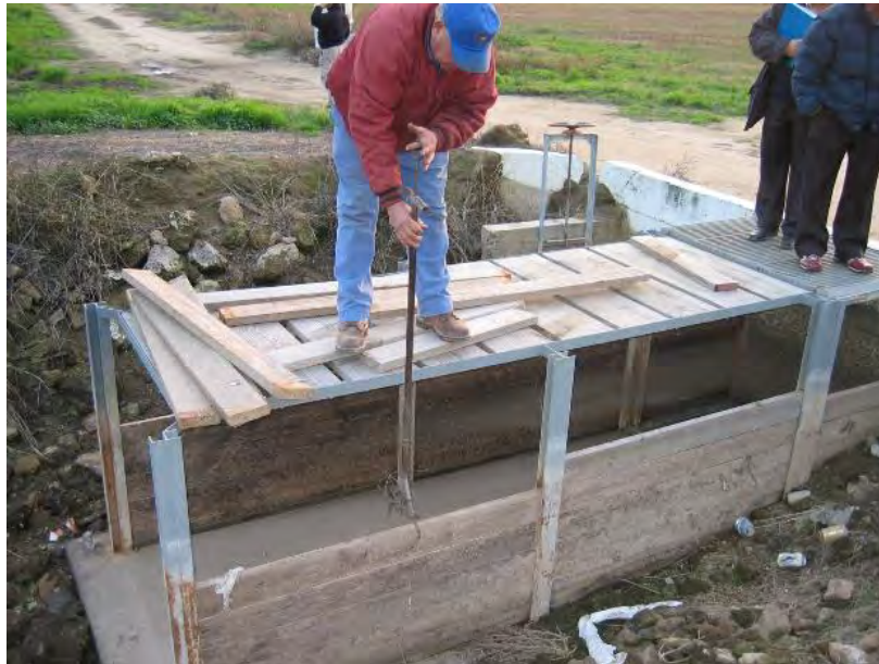
Figure 14. Example of a simple structure with slots for flashboards
