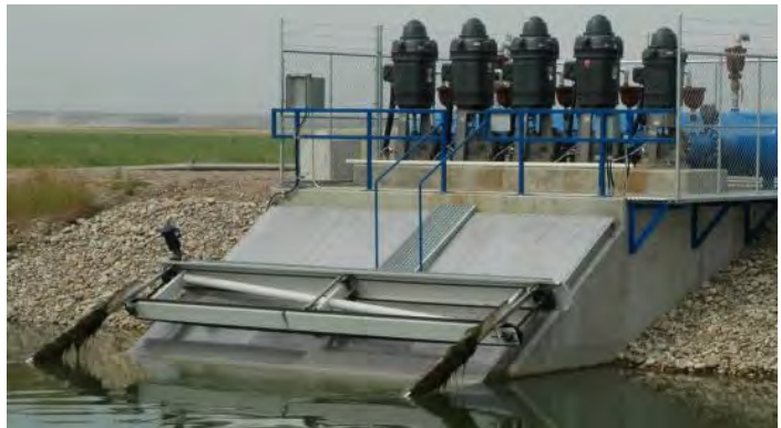
Figure 54. Self-sweeping screen and trash rack cleaner manufactured by Aqua Systems 2000 Inc.
