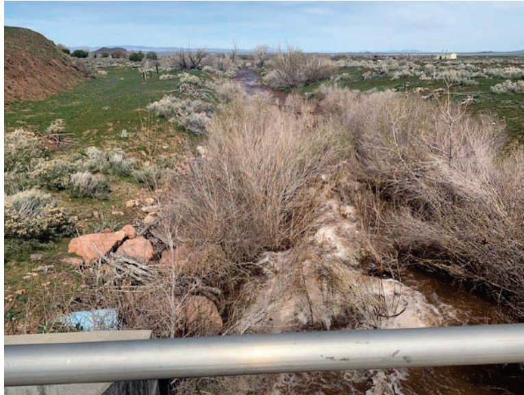
Caption: Willow growth in outlet discharge channel.
