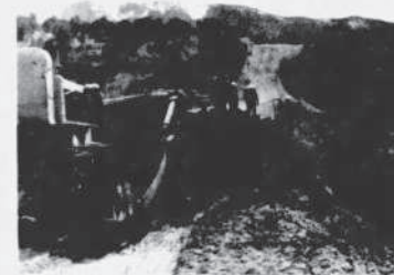
Workers rock to dump dirt and rock into area of dam that was breaking off. Water at the center-right of photo is coming from break in dam.
