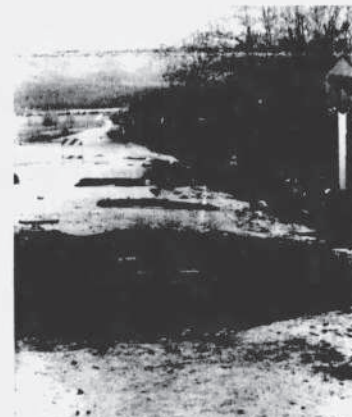
Street at the south end of town was breached and canal widened to keep water from flowing north down Main Street.
