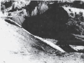
A large gap in the Kanosh Dam was left after reservoir water undermining it had been seeping through the spillway wing wall for a couple of weeks and finally collapsed this portion of the dam.
