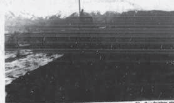
Only one lane of traffic is left on which to enter or leave town. The floodwaters ate away half the road north of Kanosh Friday night before workers could divert some of the water to the road's ditch.
