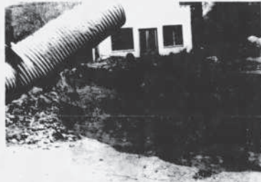
Culvert on road at south end of town could not carry all the water and was removed so channel could be widened to prevent flooding of Kanosh streets and homes.
