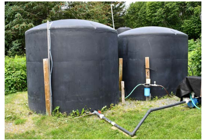
Depending on the design, tanks may be needed to temporarily store water for irrigation.
