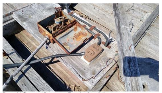
Figure 26. Destroyed Pumphouse Electrical Installation
