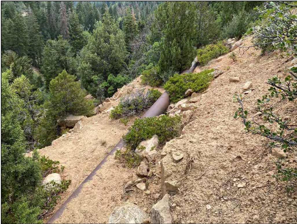
Photograph 4: Northwest view of pipeline route on southeastern portion of Action Area
