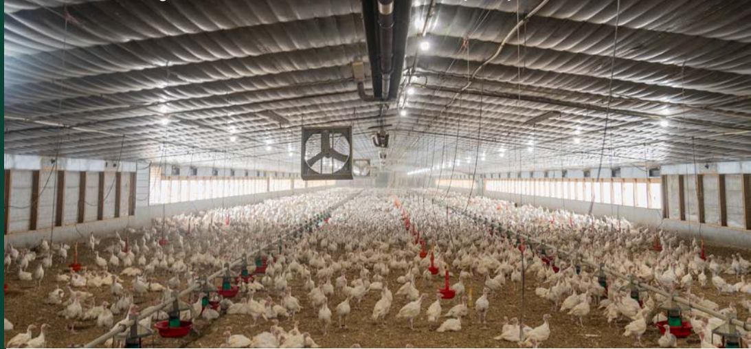
New radiant heating and barn insulation in one of John Baker's poultry barns.
