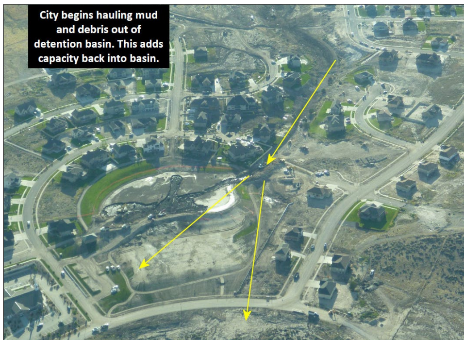
Figure E-5 Sediment-laden flow through residential neighborhood
