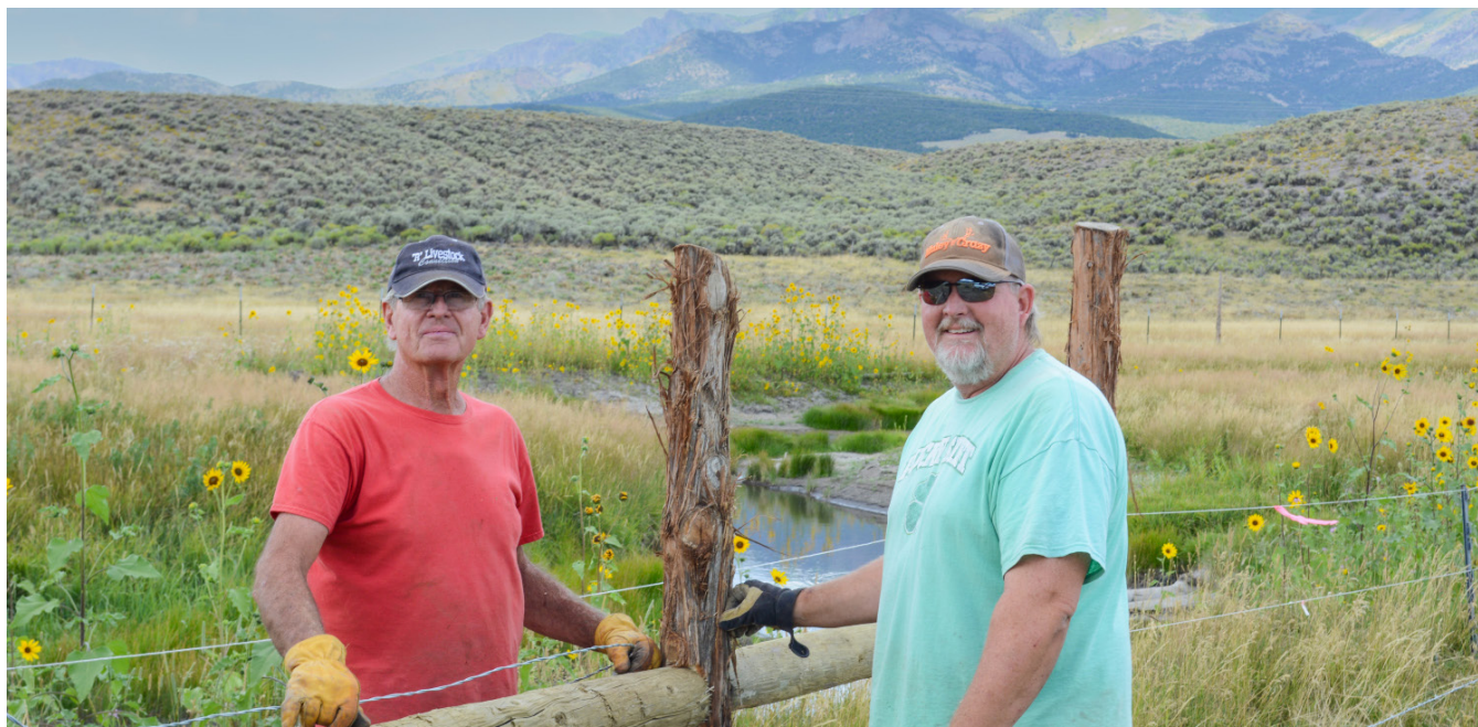
This father and son team has been working with the Utah PFW program for several years improving in-stream, wetland, riparian, and upland habitat. Here they are constructing fence for a riparian pasture along Otter Creek in southern Utah. Relationship building is one of the unmeasurable aspects of PFW program projects. Photo by Clint Wirick, USFWS.
