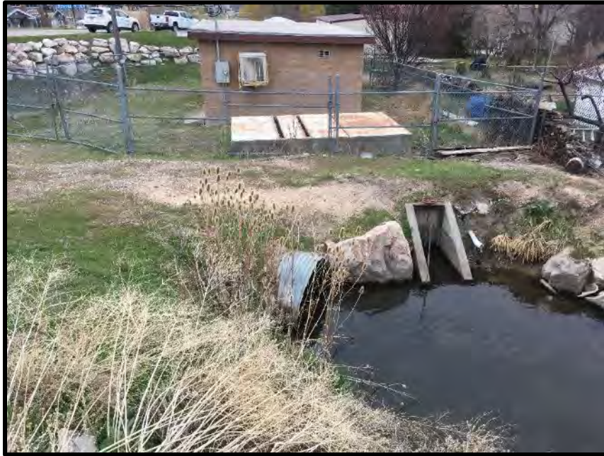
Photo 1: The beginning extent of Site 1, the North Ogden Canal existing pump station, is depicted in this photo. At this point, irrigation water enters the pipeline that would be replaced as part of the project. The pump station would be updated as well.
