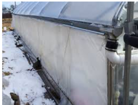
Roof runoff structure /High Tunnel
