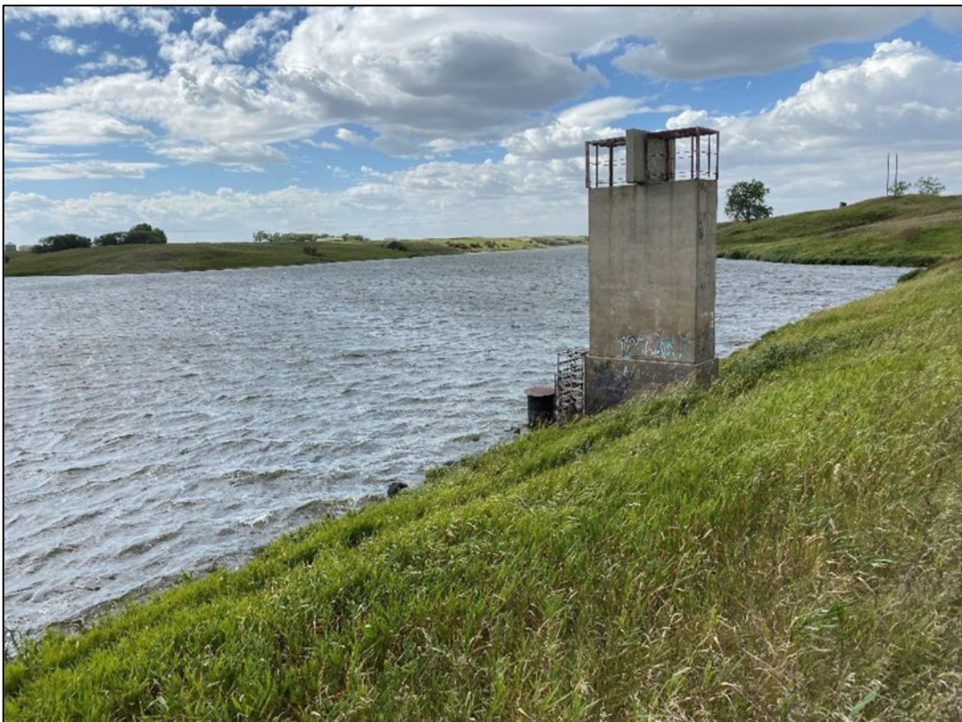
Figure 33: Primary spillway riser tower for Bylin Dam, looking west.
