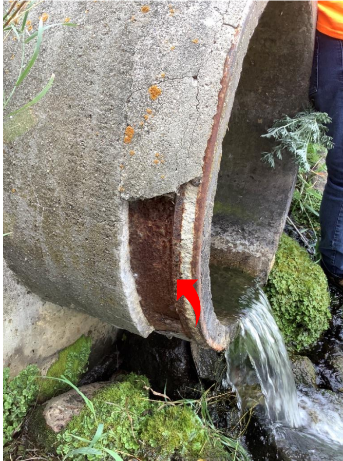
18. PRINCIPAL SPILLWAY OUTLET CONCRETE LOSS
