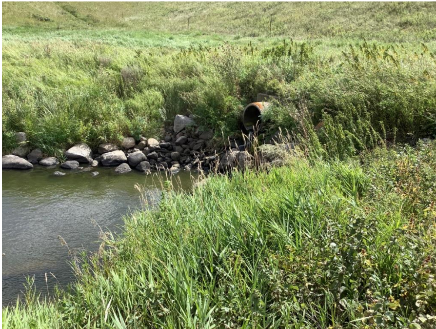
16. PRINCIPAL SPILLWAY OUTLET
