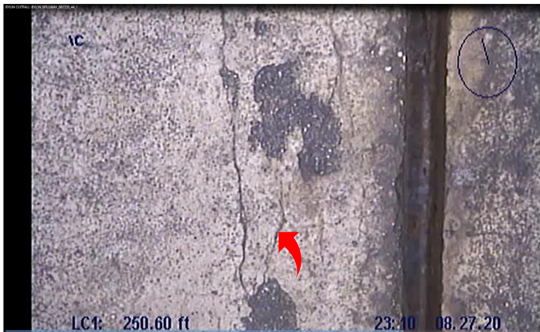
15. PRINCIPAL SPILLWAY CONDUIT PIPE CRACK (NEAR JOINT 11)
