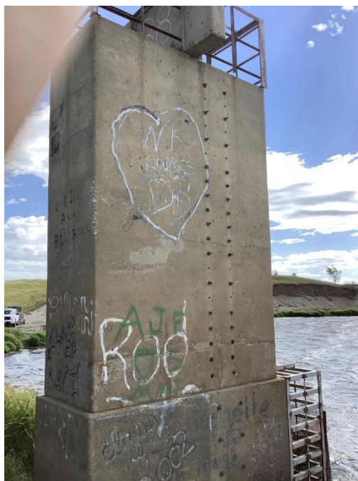
6. MINOR SPALLING NORTHEAST CORNER OF RISER
