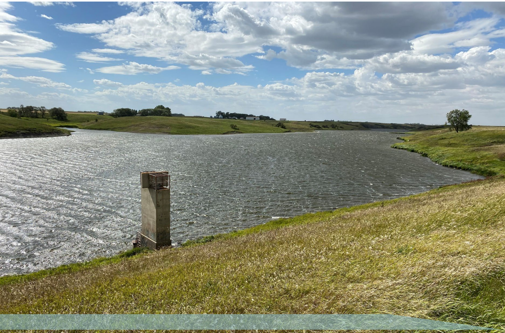
Principal Spillway Riser Tower and Reservoir at Bylin Dam – Walsh County, North Dakota
