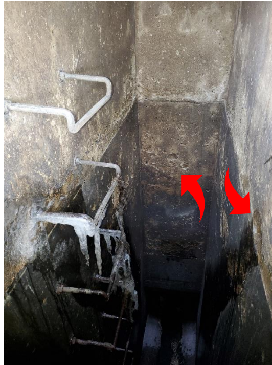
9. INTERIOR RISER MINOR SPALLING (LOOKING EAST)
