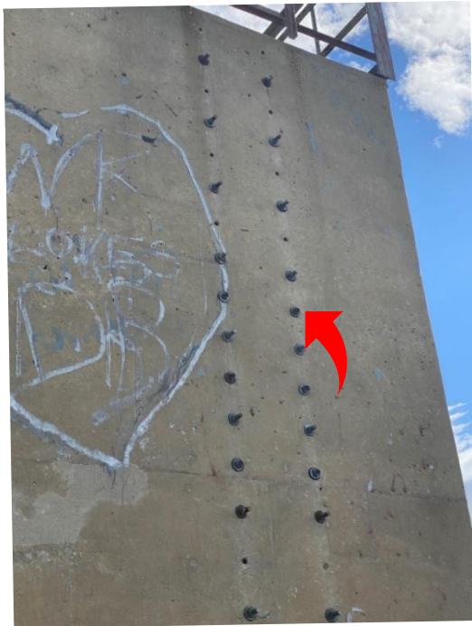
7. OPEN ANCHOR HOLES (NORTH RISER FACE)
