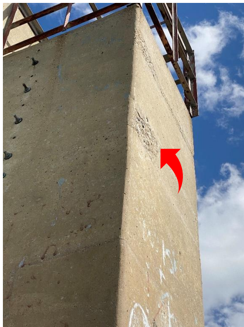
3. MINOR SPALLING WEST FACE OF RISER
