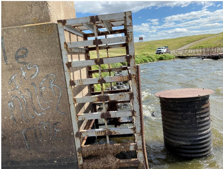
1. THRASH RACK & CAPPED VALVE WELL (FRONT OF RISERS)
