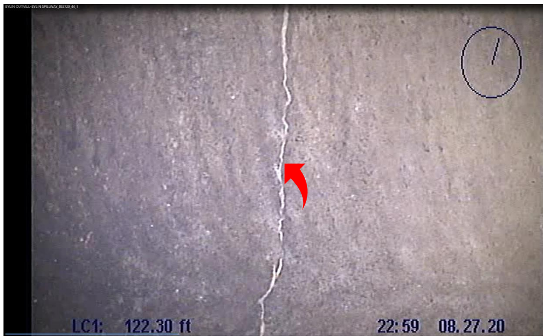
14. PRINCIPAL SPILLWAY CONDUIT PIPE CRACK (NEAR JOINT 4)
