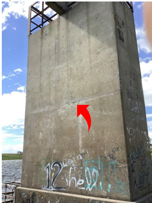
5. MINOR SPALLING SOUTH FACE OF RISER
