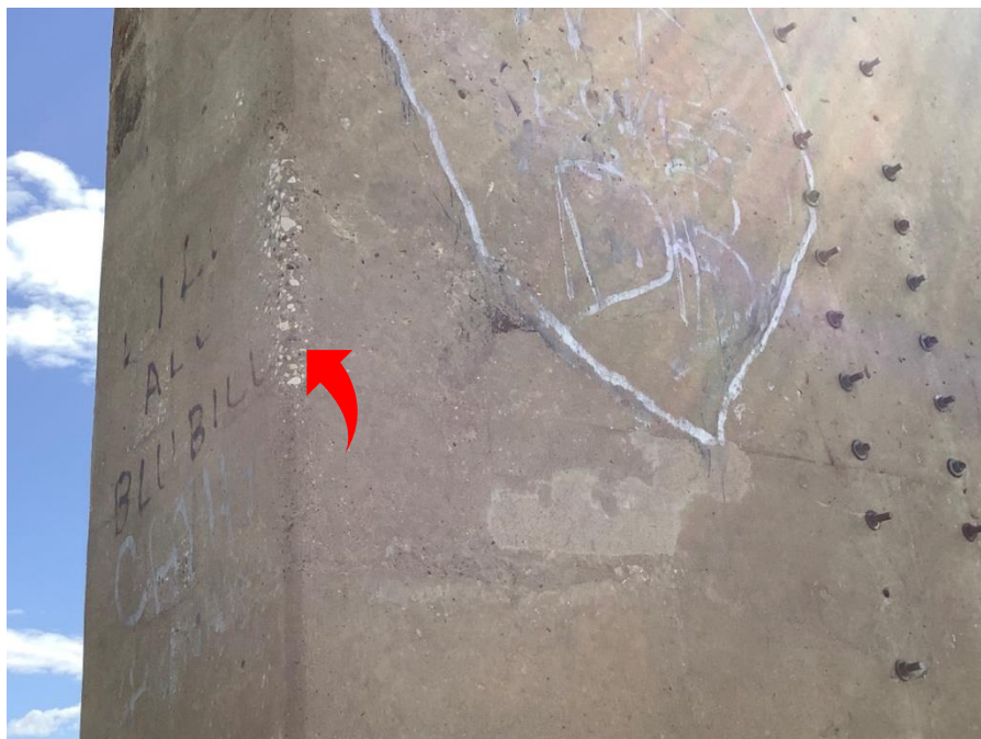
4. MINOR SPALLING NORTHEAST CORNER OF RISER
