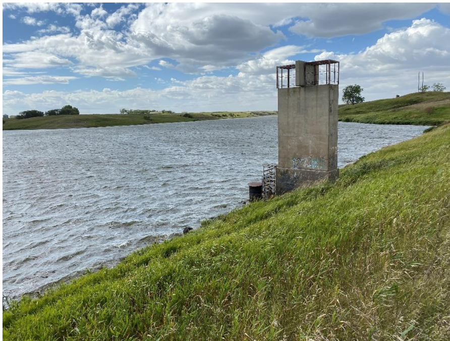
2. PRINCIPLE SPILLWAY RISER STRUCTURE
