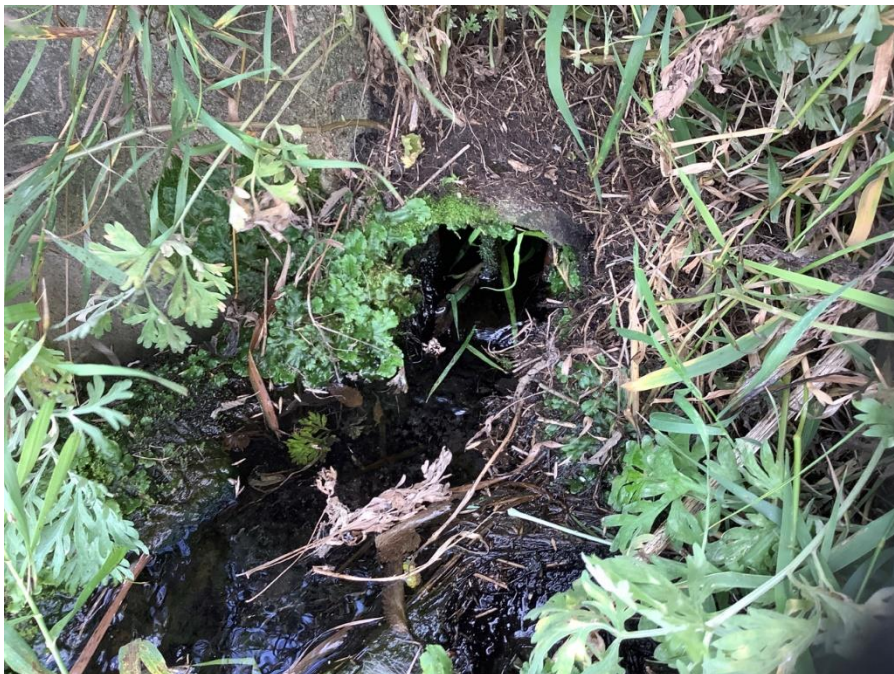
13. LEFT (NORTH) FOUNDATION DRAIN (MISSING RODENT SCREEN)
