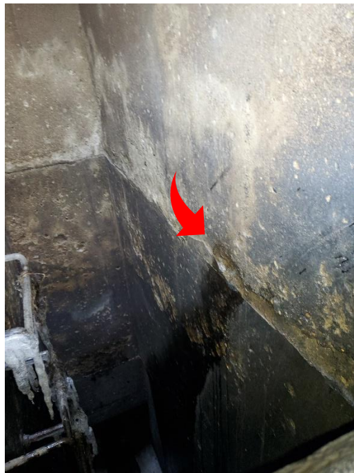
10. INTERIOR RISER MINOR SPALLING (SOUTH WALL)
