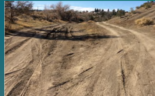
Looking up auxiliary spillway
