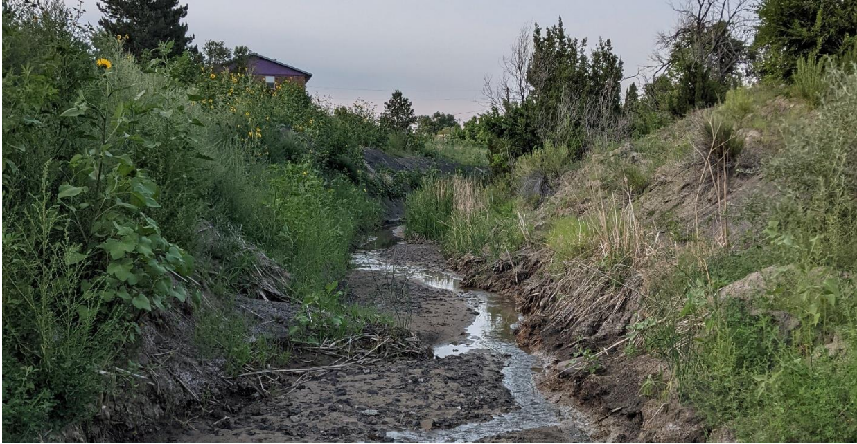
Figure 1. Channel immediately downstream of dam outlet exhibiting minimal riparian vegetation
