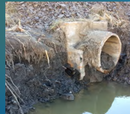
Principal Spillway Outlet
