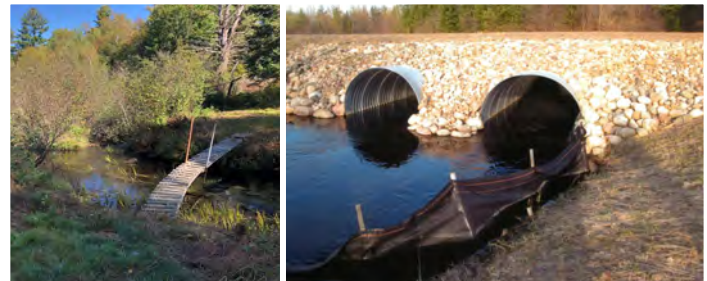
Before and after photos of the stream crossing location.
