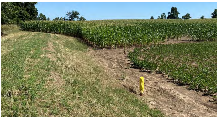
Part of Water and Sediment Control Basin (WASCOB) installed.
