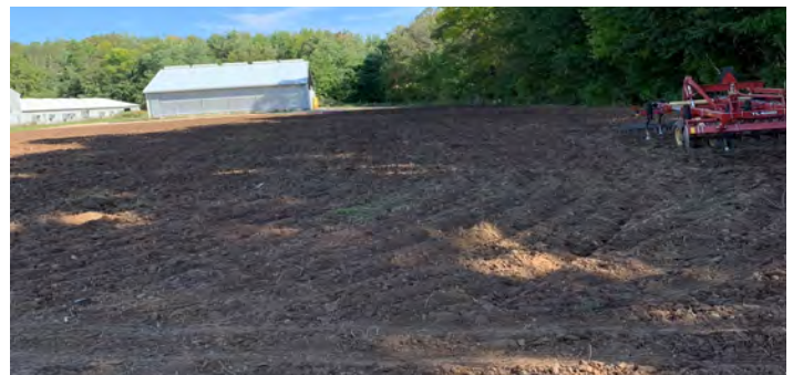
Finished grade over the closed manure storage facility site.
