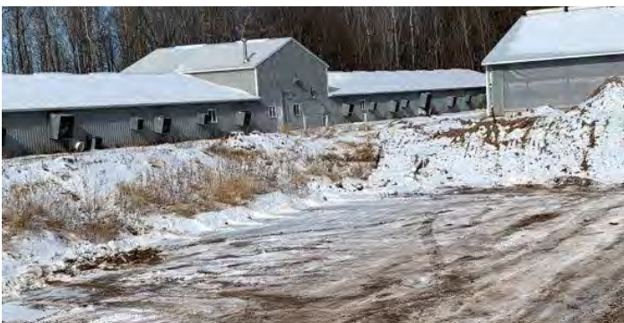
Former manure storage facility ready for closure.
