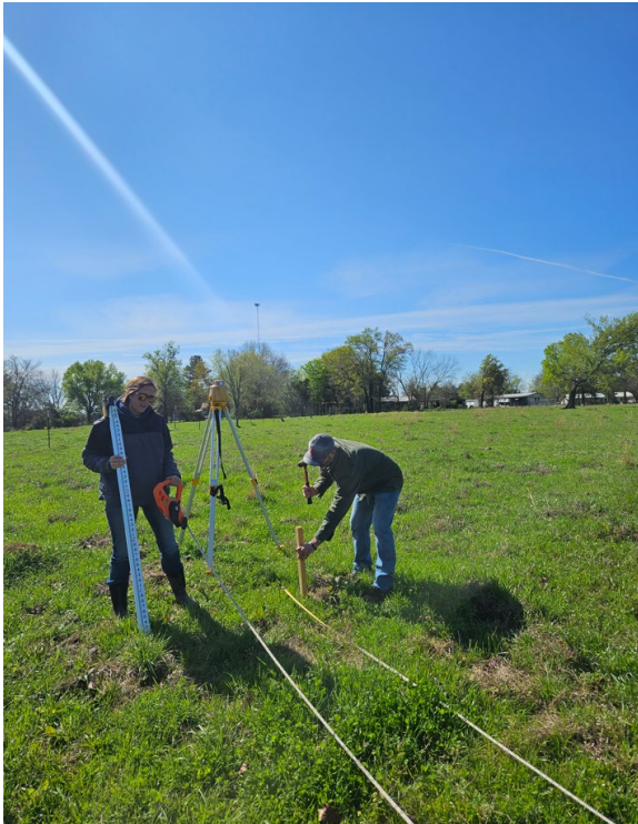
Figure 1.—Using a laser level to set up slope stakes.
