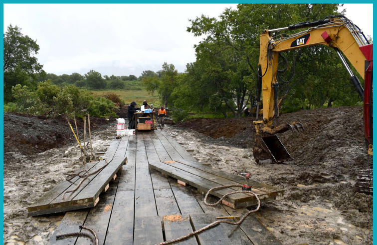
Constructing a mud sill boardwalk.
