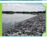
Treatment used to stabilize and protect banks of streams or constructed channels and shorelines.
