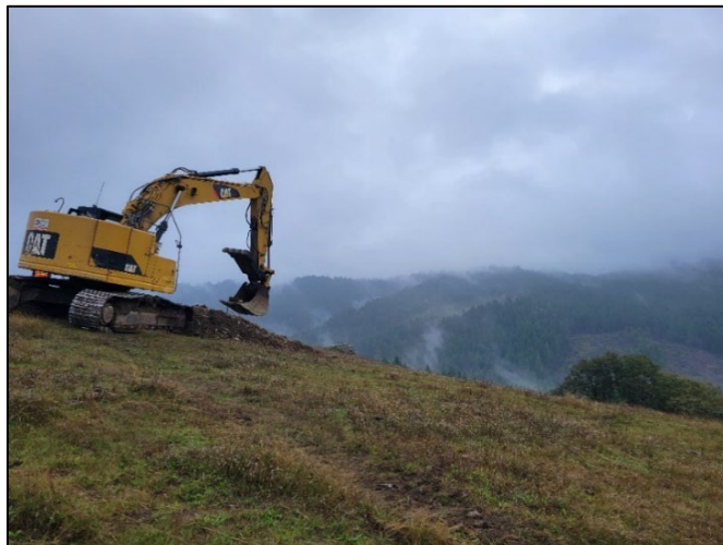
Figure 3. —An excavator digging one of the competition soil pits.
