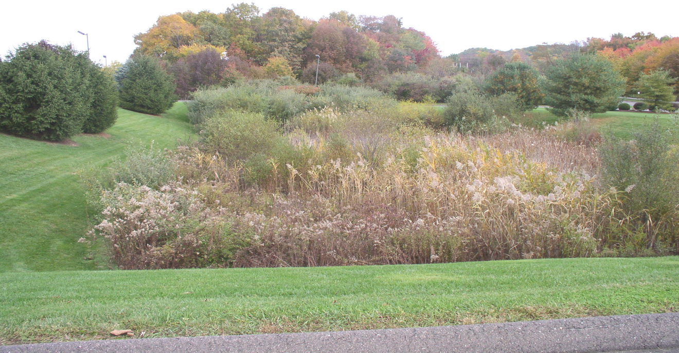
Fig. #3 Extended Detention Shallow Wetland Photo Credit: Tom Ladny, NRCS
