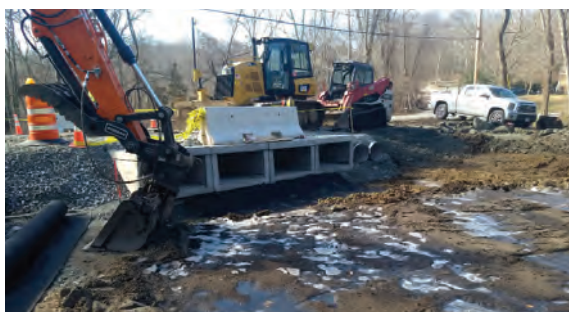
The roadway was raised to allow for safe access during flood events.
