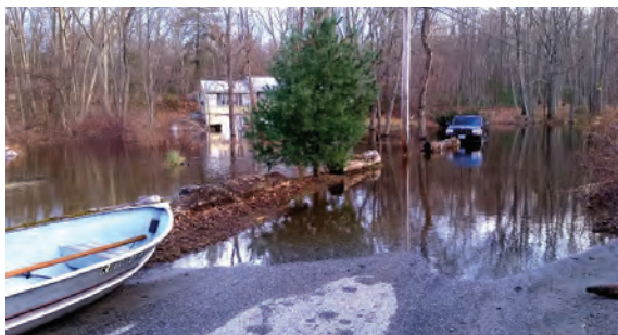
Belfield Drive experienced recurrent flooding from the Pocasset River that made the road impassible.
