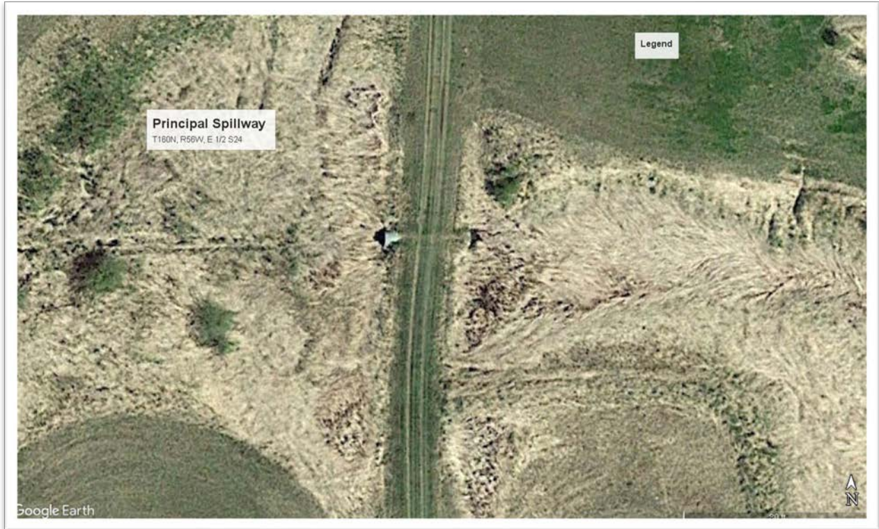
Figure 23. Extant structure and flood zone at proposed principal spillway. Image: Google Earth 2019.
