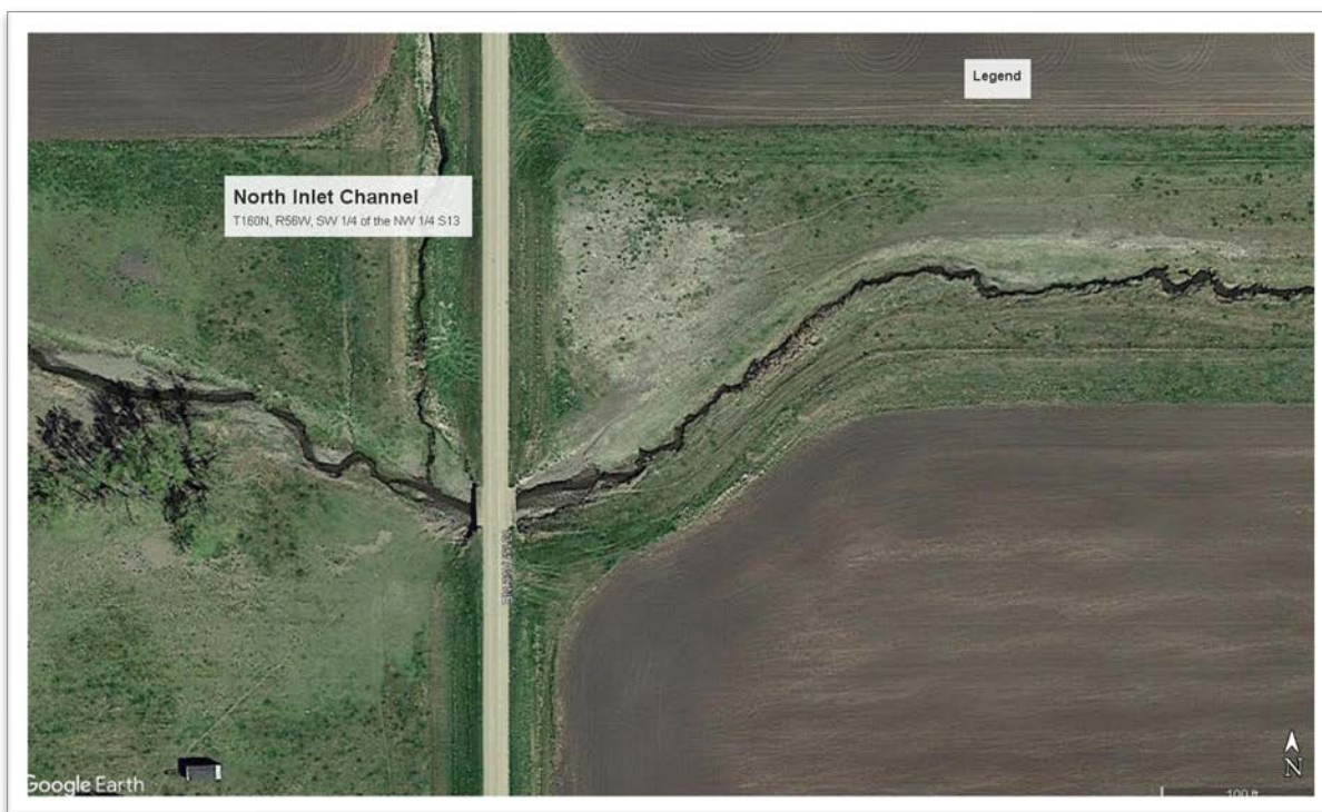
Figure 22. Extant structure at proposed north inlet channel. Image: Google Earth 2019.
